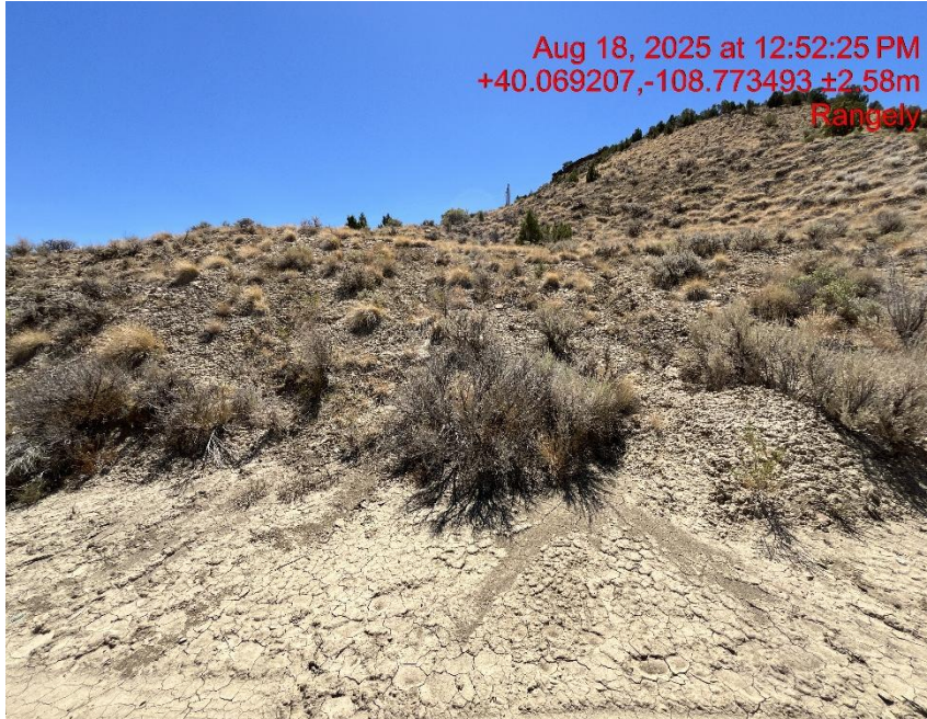
Photo # 2118 Failure to minimize erosion & transport of sediment onto location/insufficient BMP's
