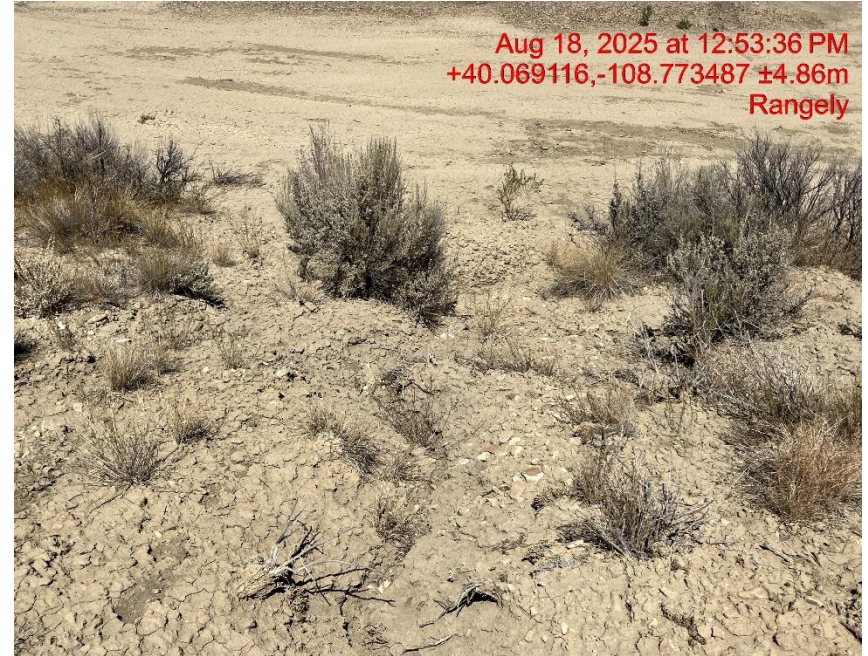
Photo # 2119 Failure to minimize erosion & transport of sediment onto location/insufficient BMP's
