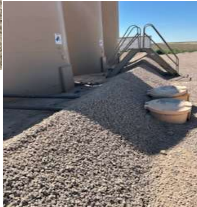
Burrows in Berms Repaired
