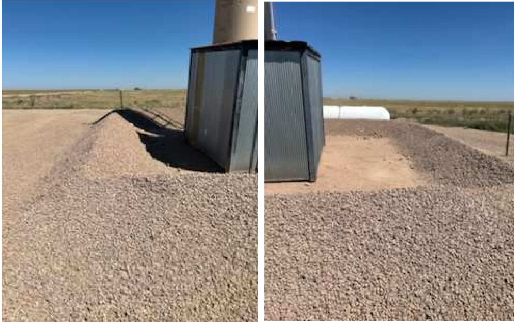
Burrows in Berms Repaired
