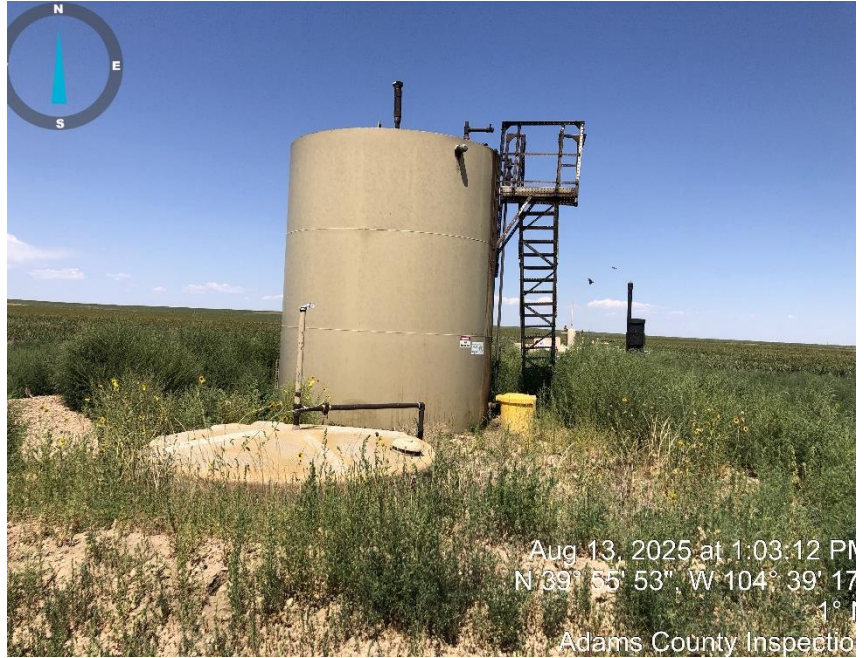
Photo #2 Tanks and weeds.
