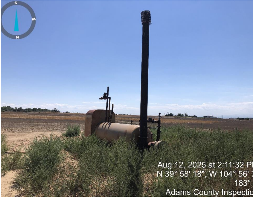
Photo #3 Separator and weeds.
