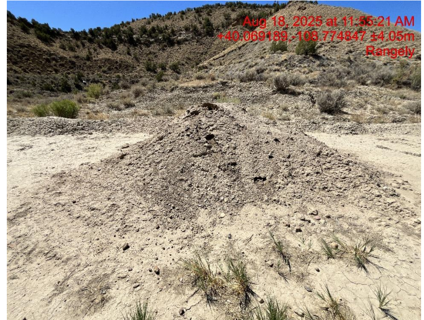
Photo # 2073 Stockpiled soils with no BMP's
