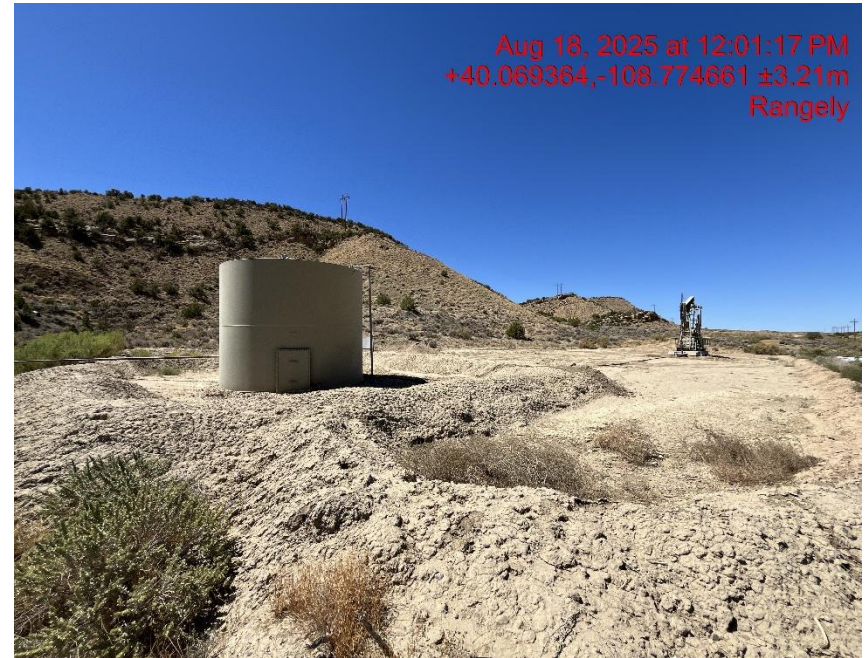
Photo # 2078 NE corner of location
