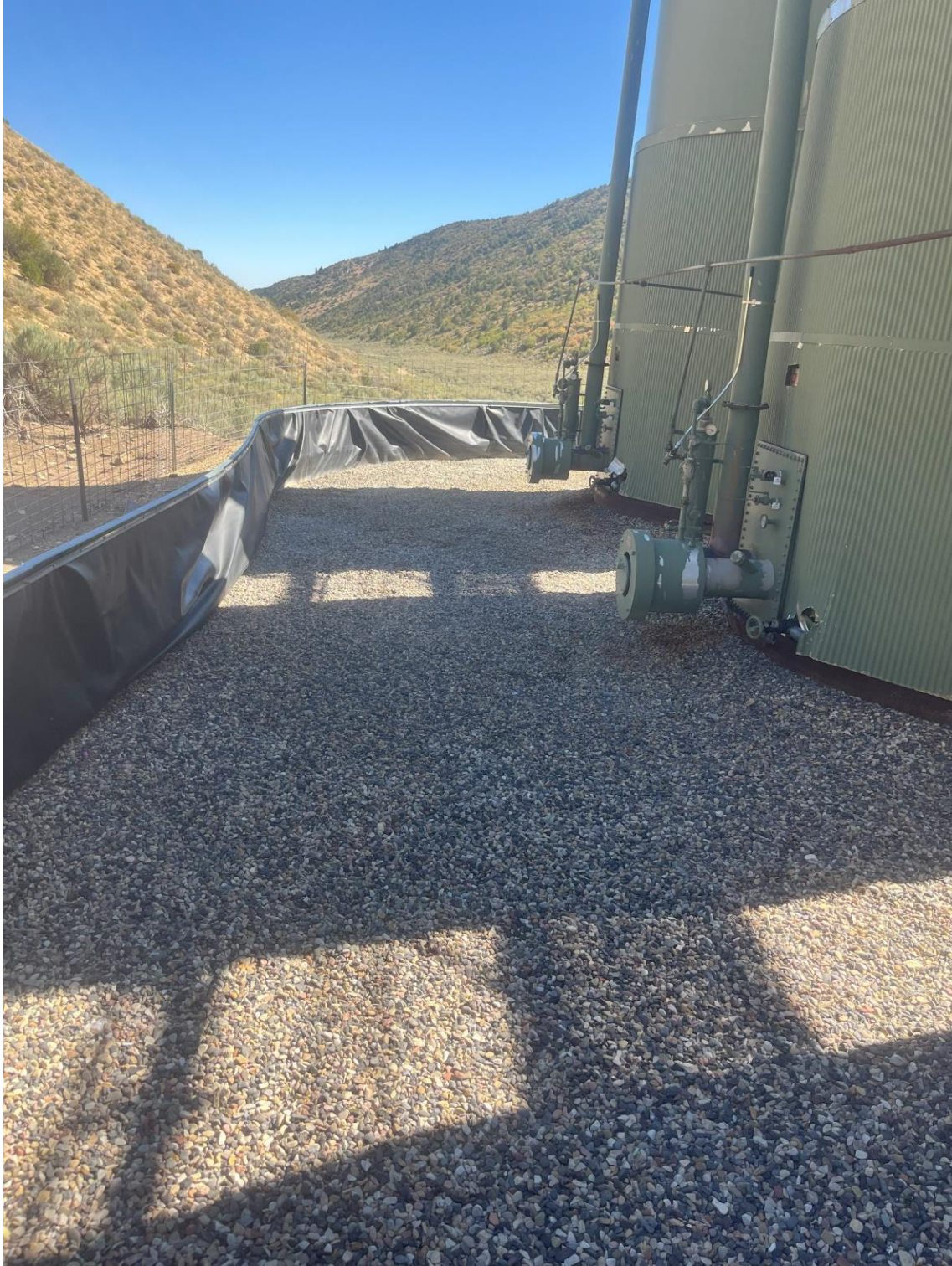
Photo of the secondary containment following fluid recovery and containment washing.
