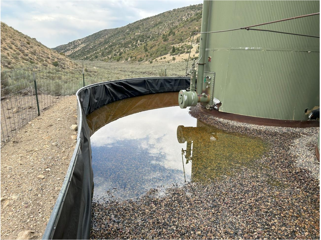
Photo of released condensate inside secondary containment.
