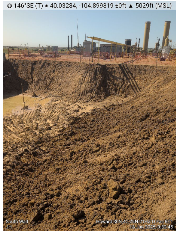
Tank Battery Excavation South Wall (Rainwater Present)
