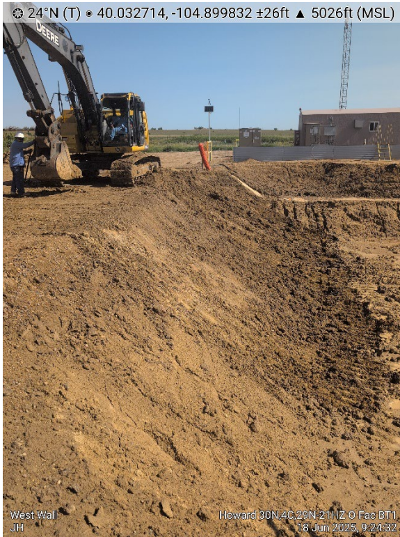
Tank Battery Excavation West Wall
