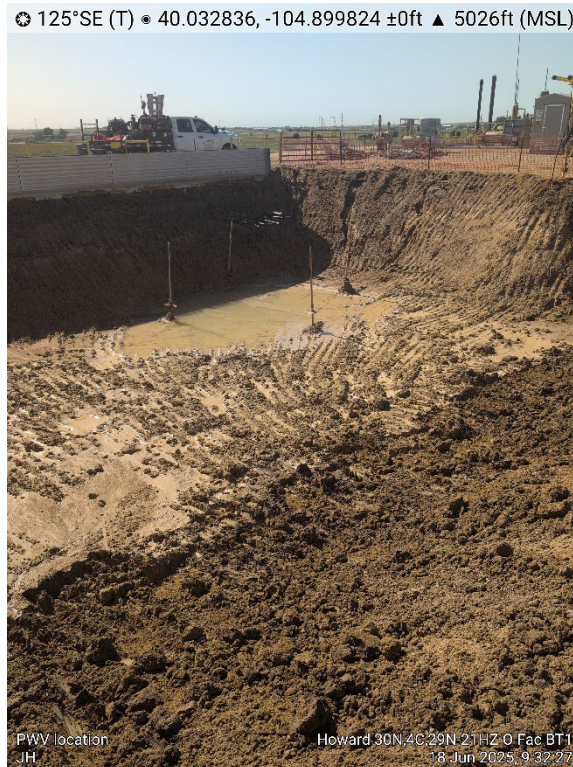
PWV Location (Rainwater Present)
