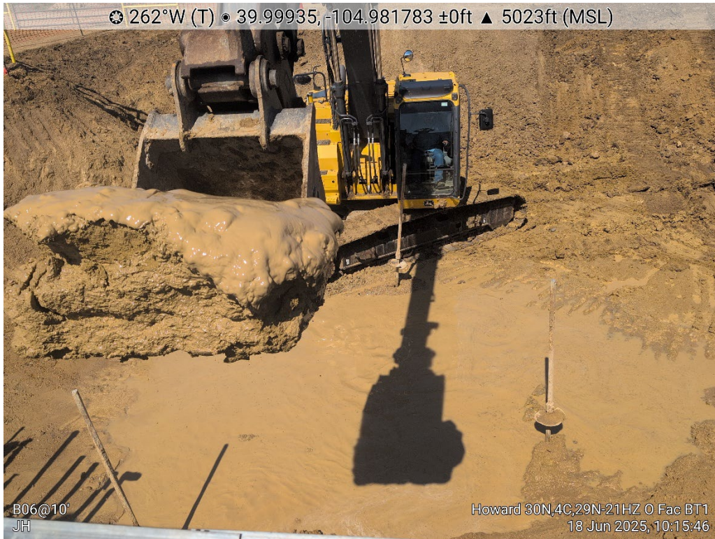
B06 Sample Location (Rainwater Present)
