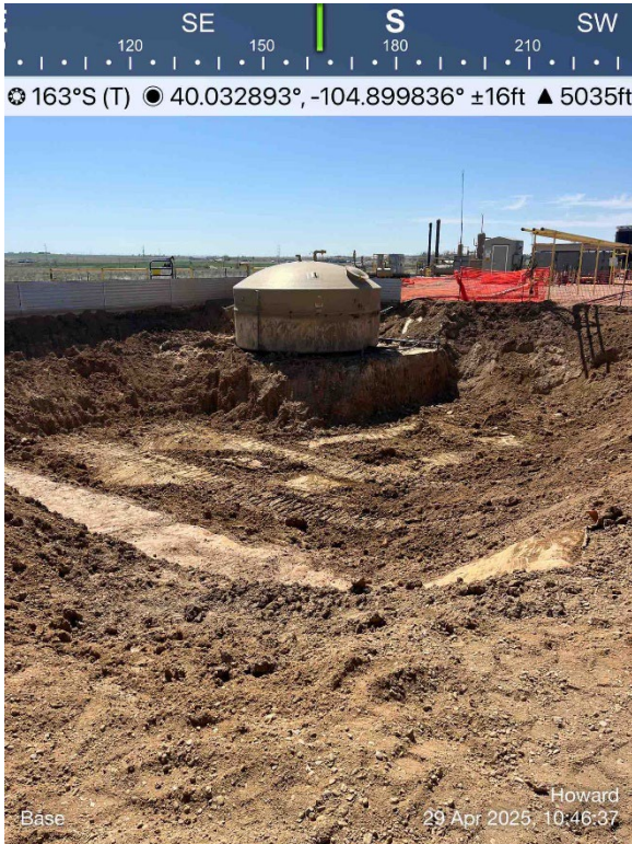
Tank Battery Excavation
