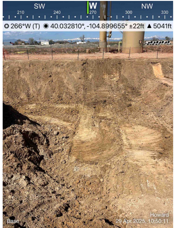
Tank Battery Excavation
