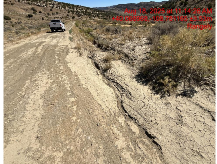
Photo # 2040 Failure to minimize erosion & transport of sediment off location/insufficient BMP's
