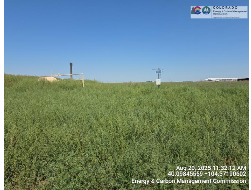
Production Equipment & Overgrown Vegetation
