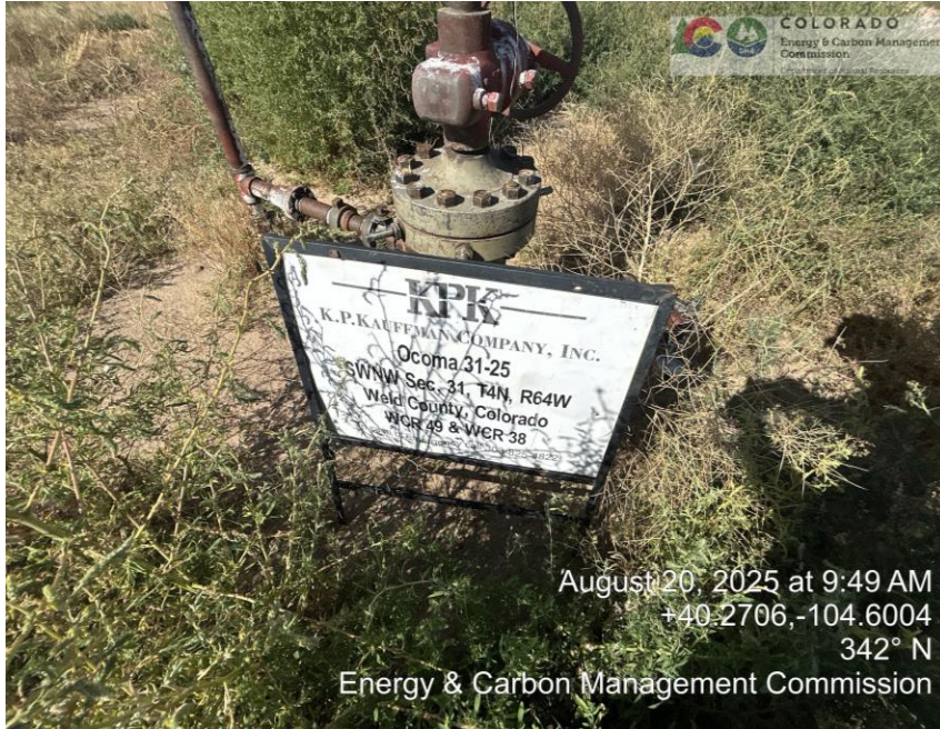
Sign & Overgrown Vegetation
