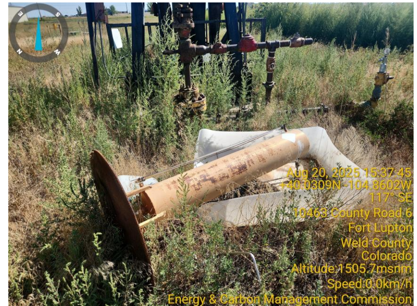
Photo 2 Wellhead overrun with tall vegetation & trash.
