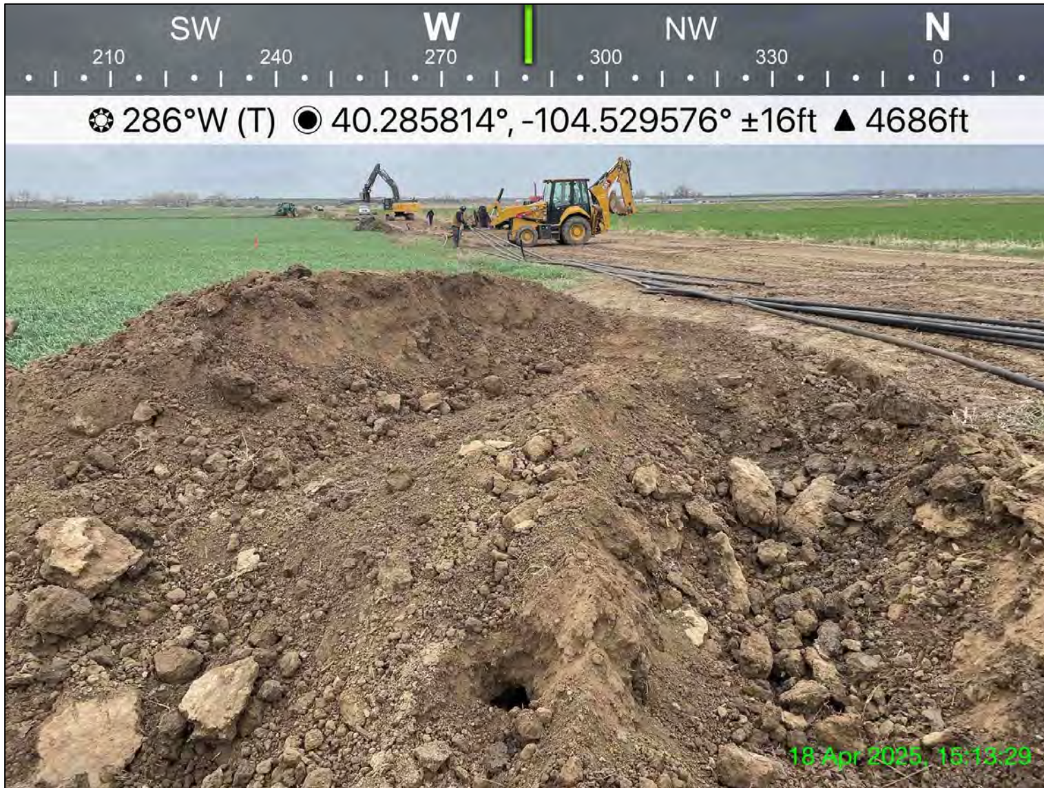
Photo 8: View of FL02-06 sampling location, facing west
