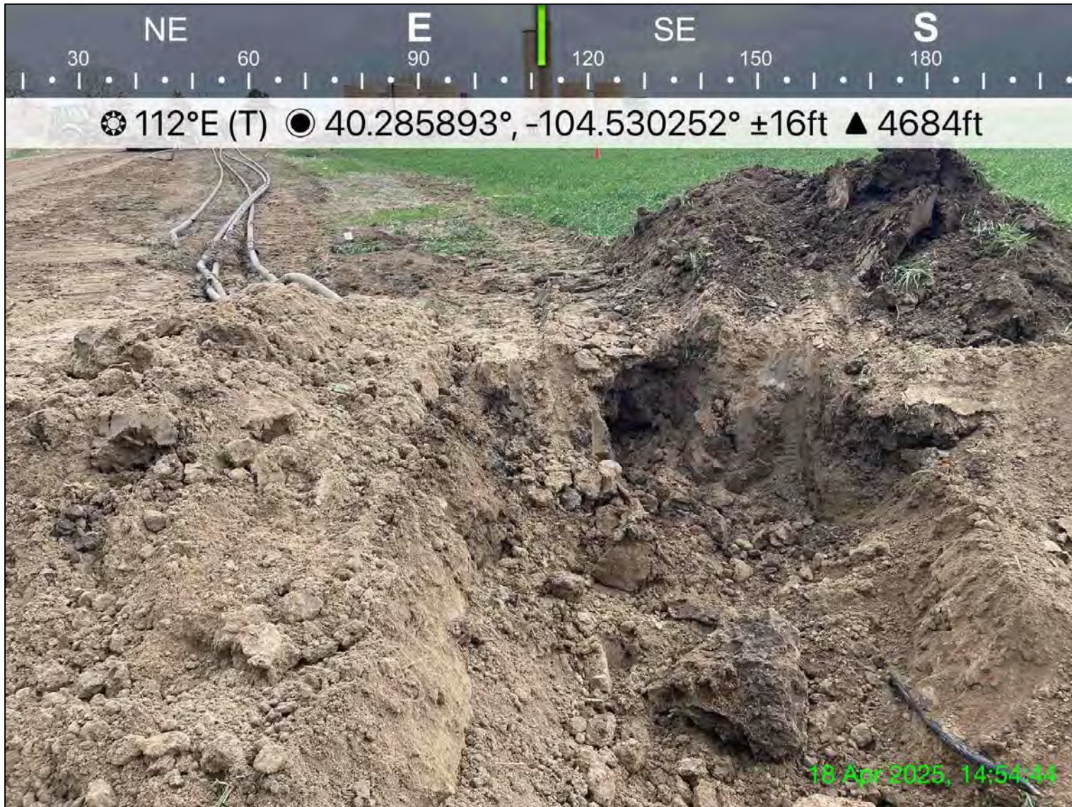
Photo 7: View of PH19 screening location, facing east
