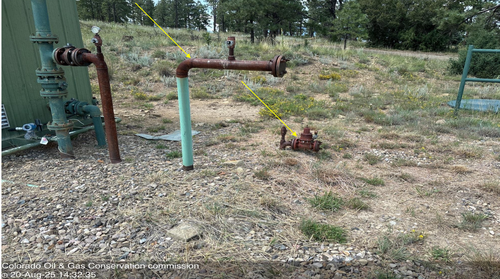
PHOTO 5: ECMC INSPECTOR FAILED TO NOTE THESE UNMARKED RISERS IN PREVIOUS INSPECTION. THESE TWO NEED TO BE MARKED WITH A PERMANENT MARKER.
