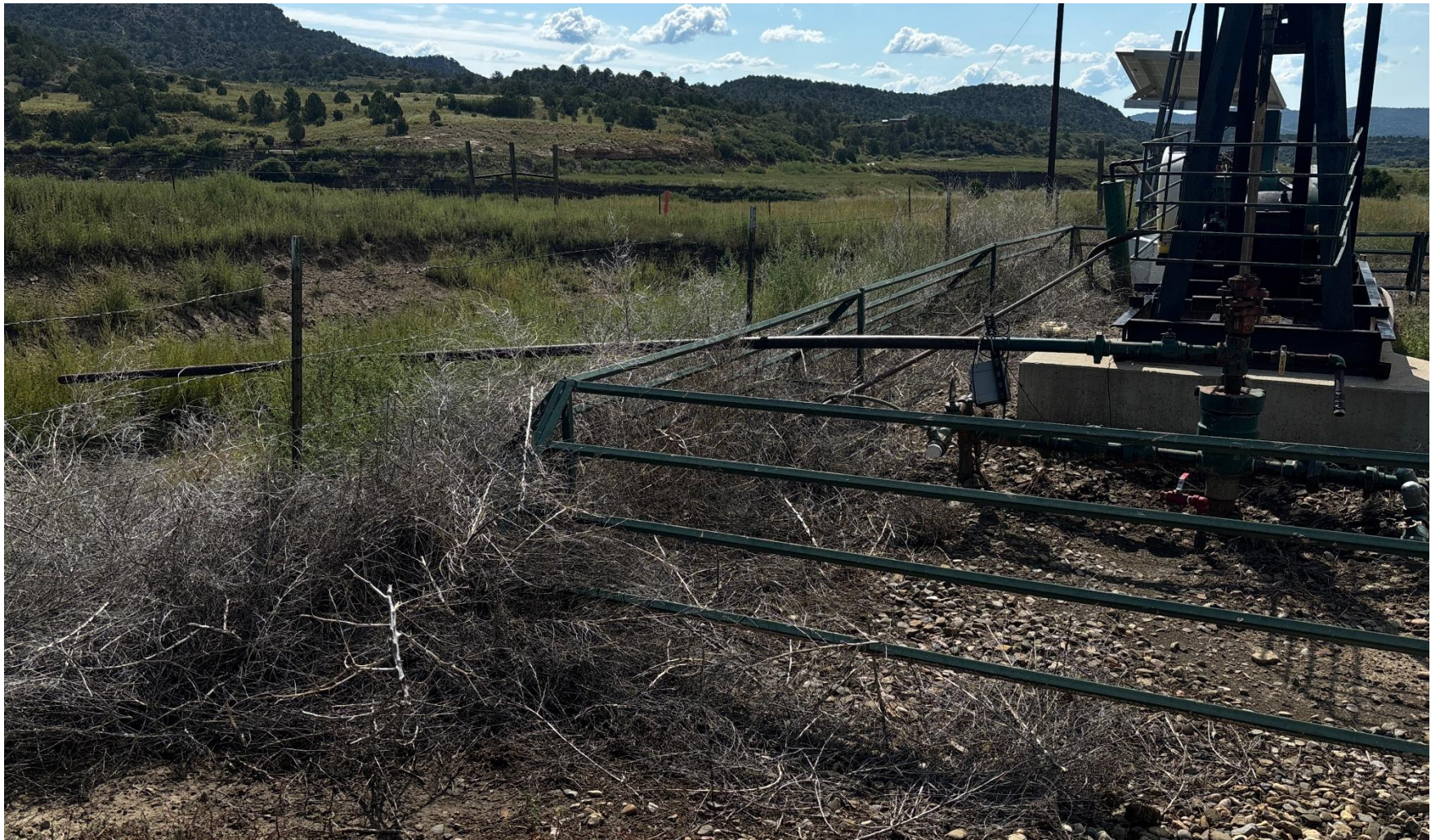
PHOTO 3: WEEDS ACCUMULATING BETWEEN PUMPJACK FENCE AND PIT FENCE. REMOVE DEAD WEEDS PER RULE 606. CA DATE 8-26-2025.
