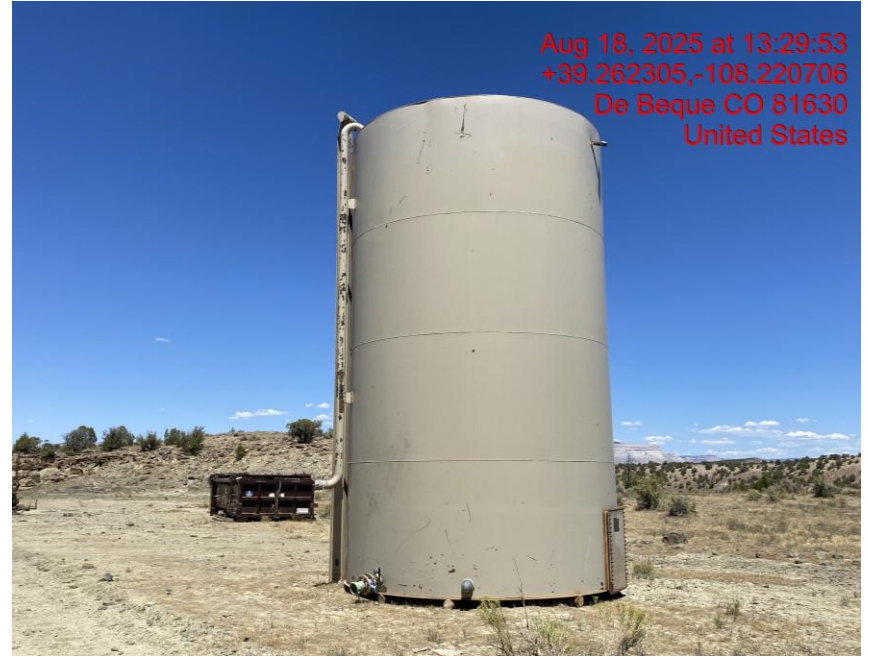
Stored Equipment – Photo #00326
