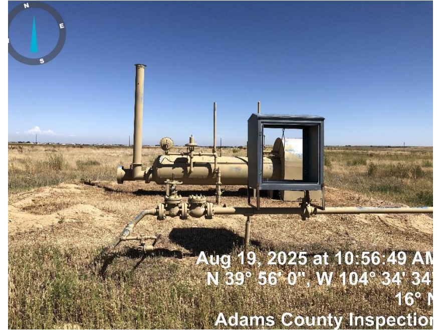
Photo#2 Separator/Gas Meter/Corrective Actions have been addressed
