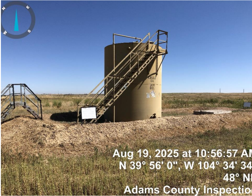
Photo#3 Production Tanks/Corrective Actions have been addressed
