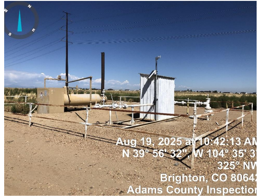
Photo#2 Separator/Gas Meter
