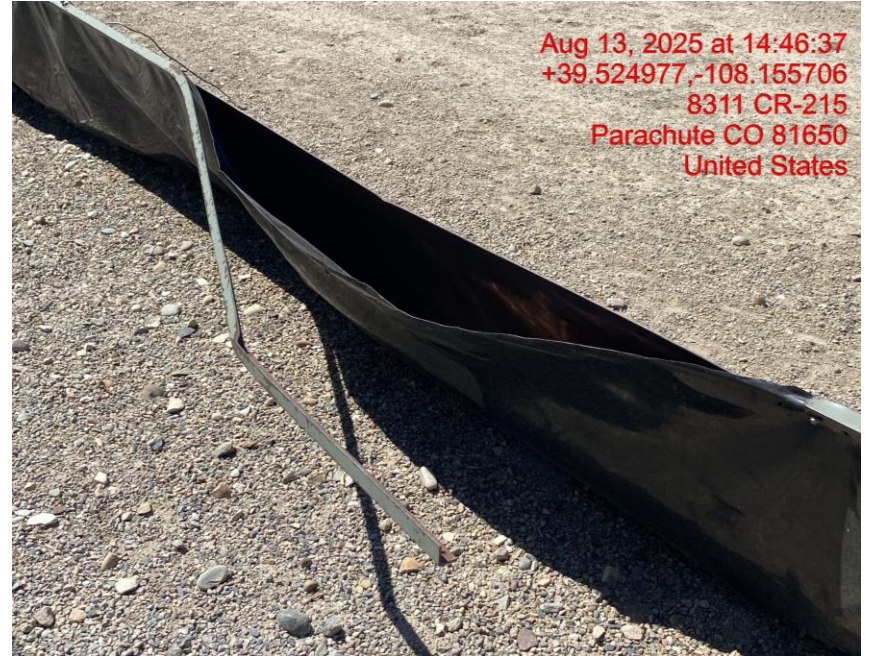
Damaged Berm – Photo #00195
