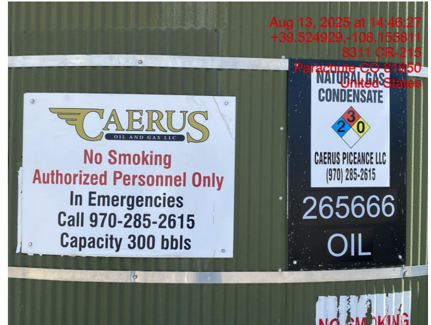
Tank Labels not Updated with Current Operator Information – Photo #00194
