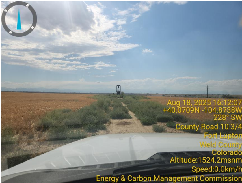
Photo 1 Access road overgrown with vegetation.
