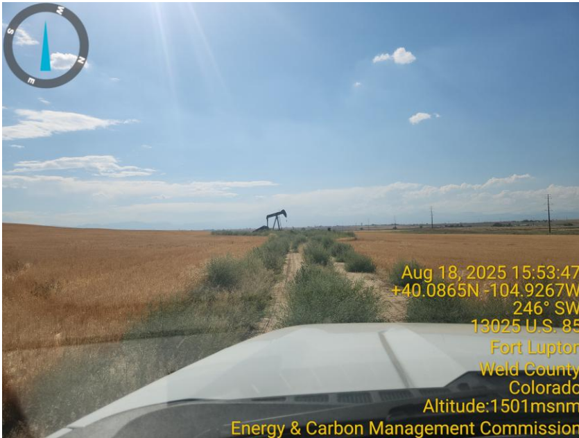
Photo 1 Access road overgrown with vegetation.
