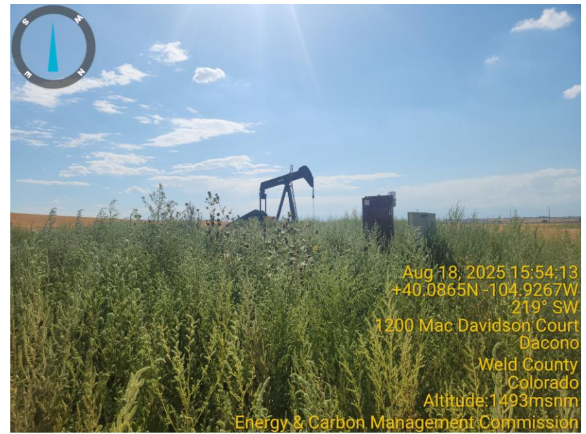
Photo 2 Ancillary equipment overrun with tall vegetation.
