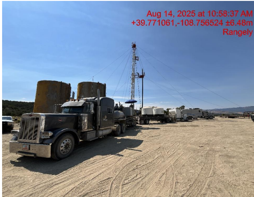
Photo # 1827 NW corner of location
