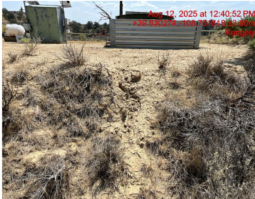
Photo # 1809 Failure to minimize erosion & transport of sediment off location/insufficient BMP's
