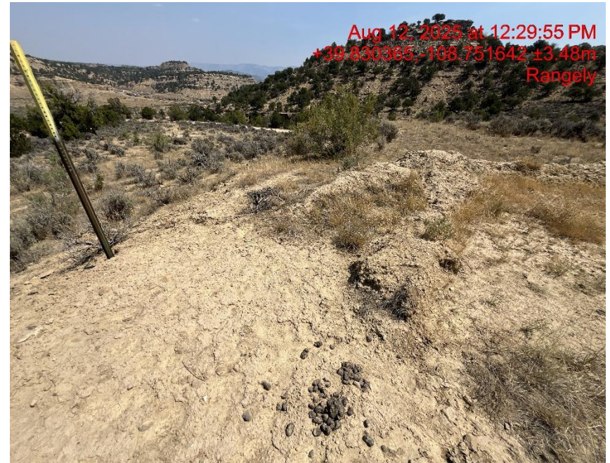
Photo # 1799 Failure to minimize erosion & transport of sediment off location/insufficient BMP's
