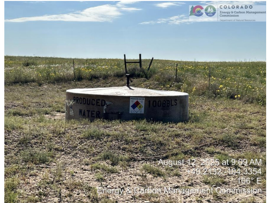
Pit/ Overgrown Vegetation
