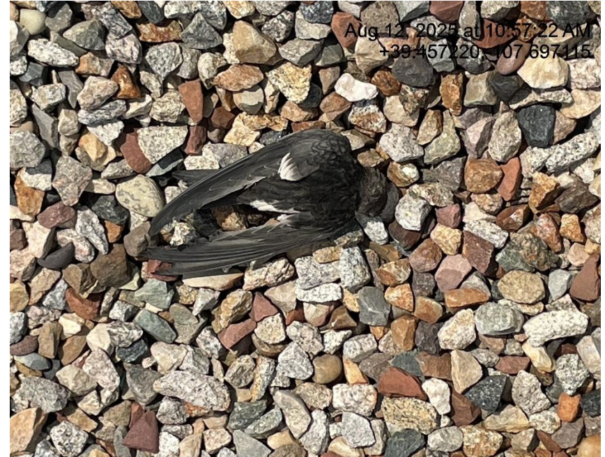
Photo # 9853 Dead bird in secondary containment
