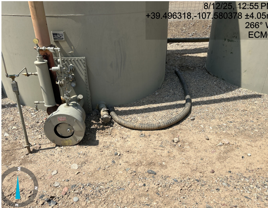
Unused hose in secondary containment
