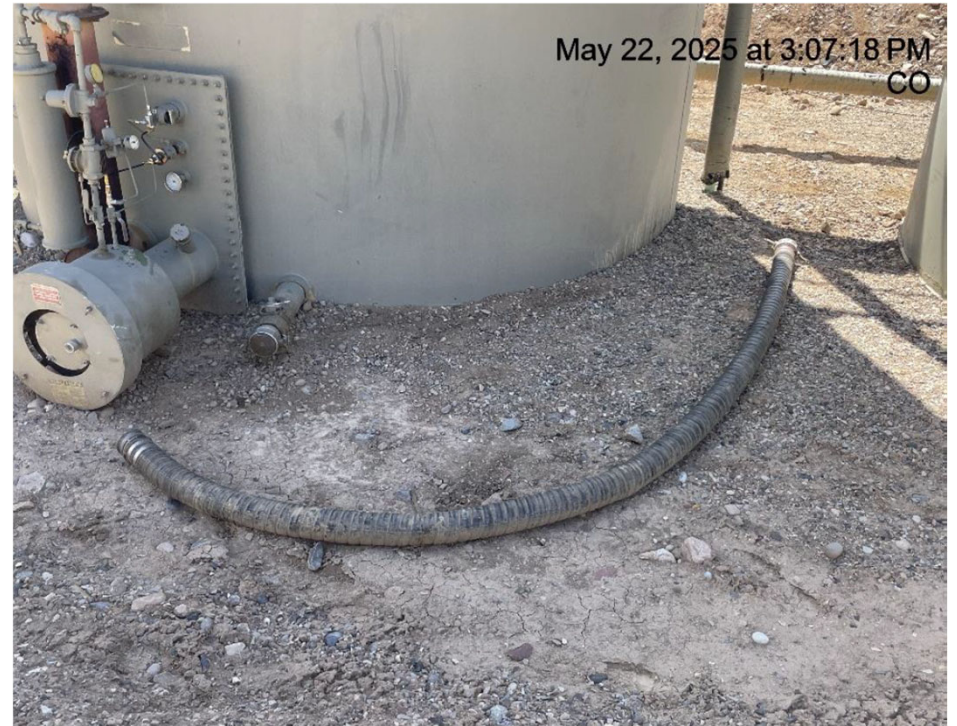
Unused hose in secondary containment (photo from previous inspection)
