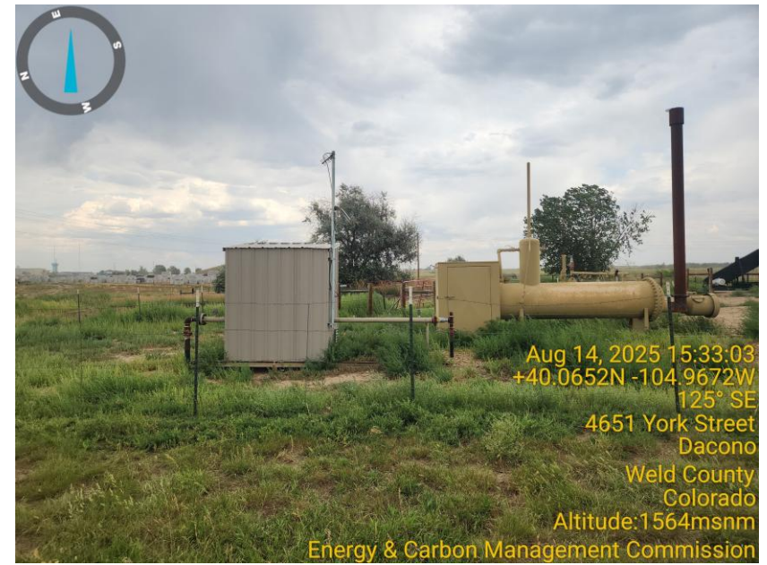
Photo 2 Gas Meter, Horizontal heated Separator.
