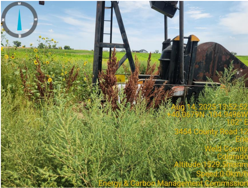
Photo 3 Wellsite Sign hidden by tall vegetation.
