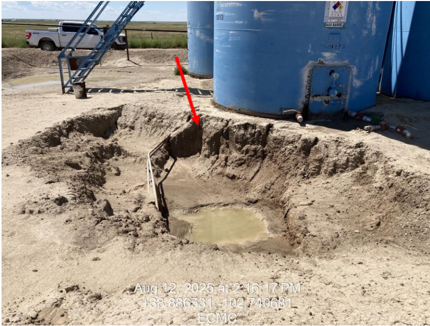
Photo 3 – Excavation within secondary containment
