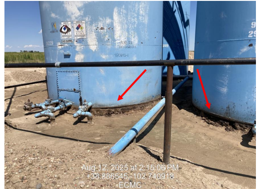
Photo 2 – Impacted material under tanks
