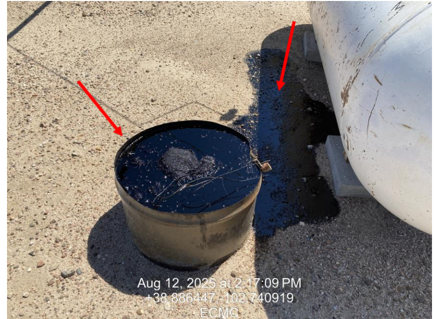
Photo 6 – Vessel with oil overflowing, impacted soils
