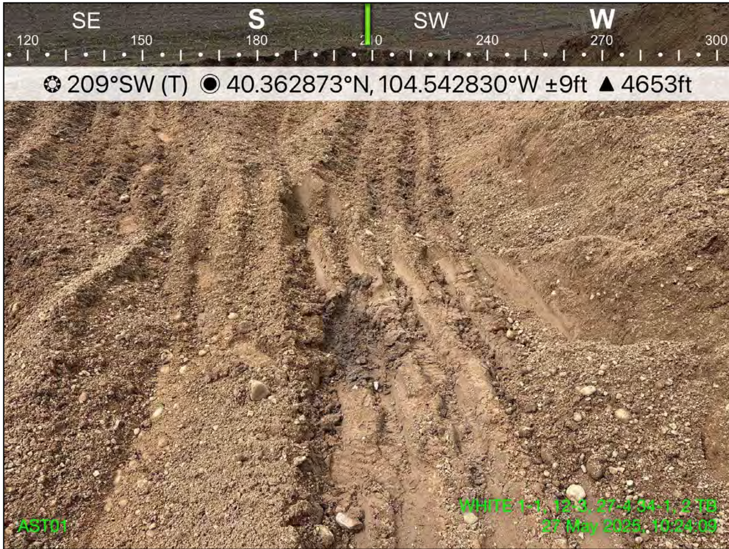
Photo 1: View of AST01 excavation area, facing southwest
