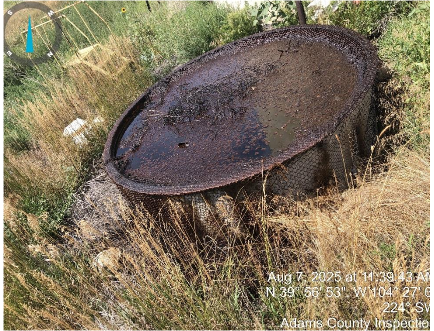
Photo #4 Open top tank flowing over.
