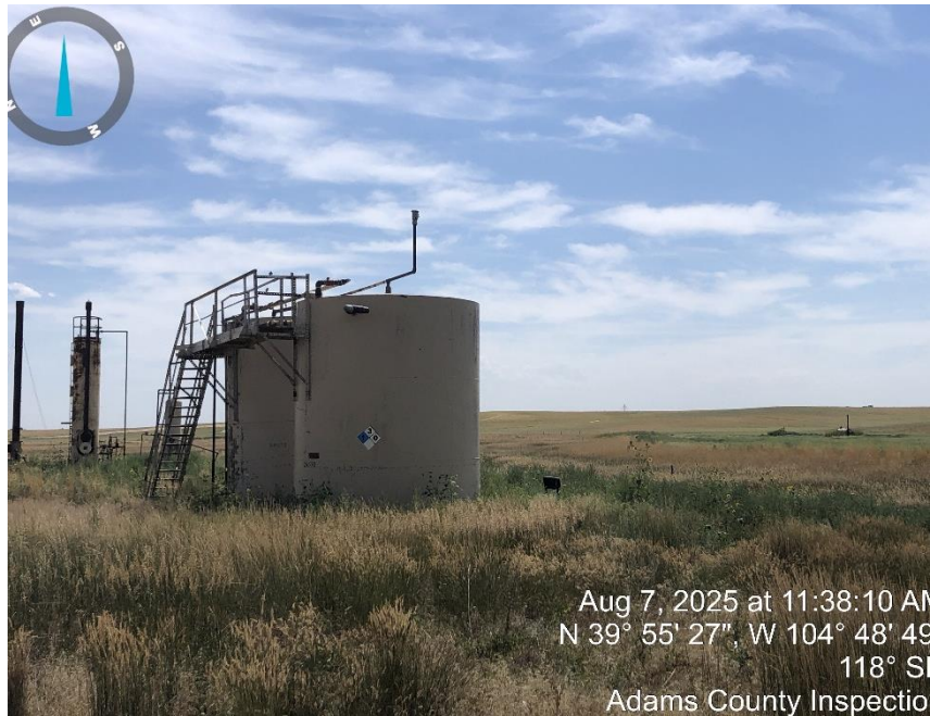
Photo #2 Tanks, separator and well head in background.
