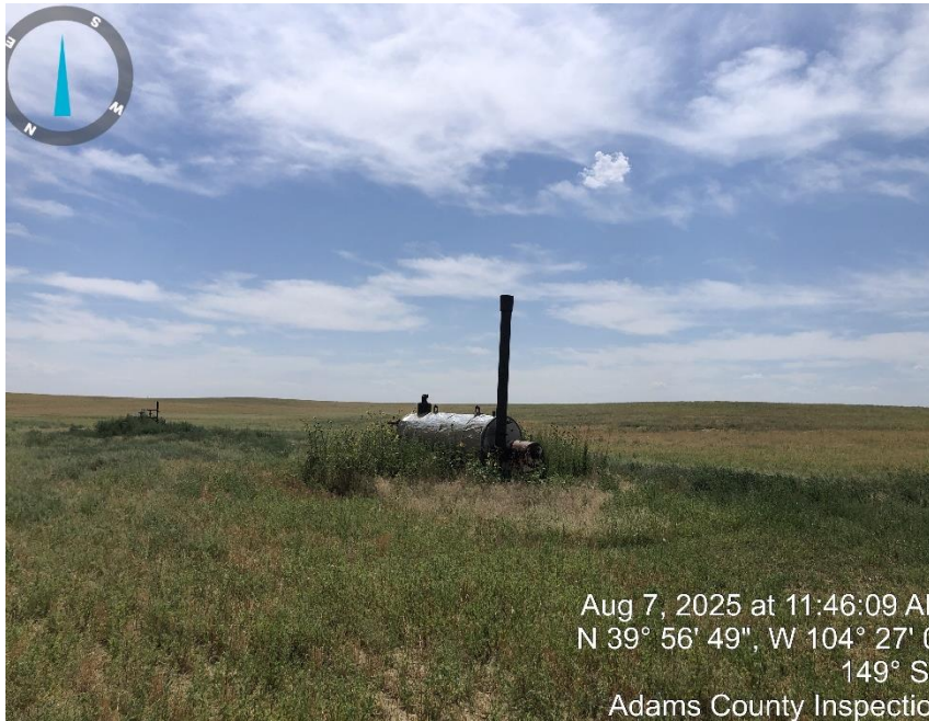
Photo #7 random separator next to well head.
