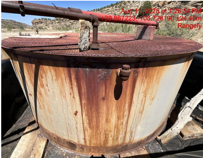
Photo # 1707 Possible leaks on production tank
