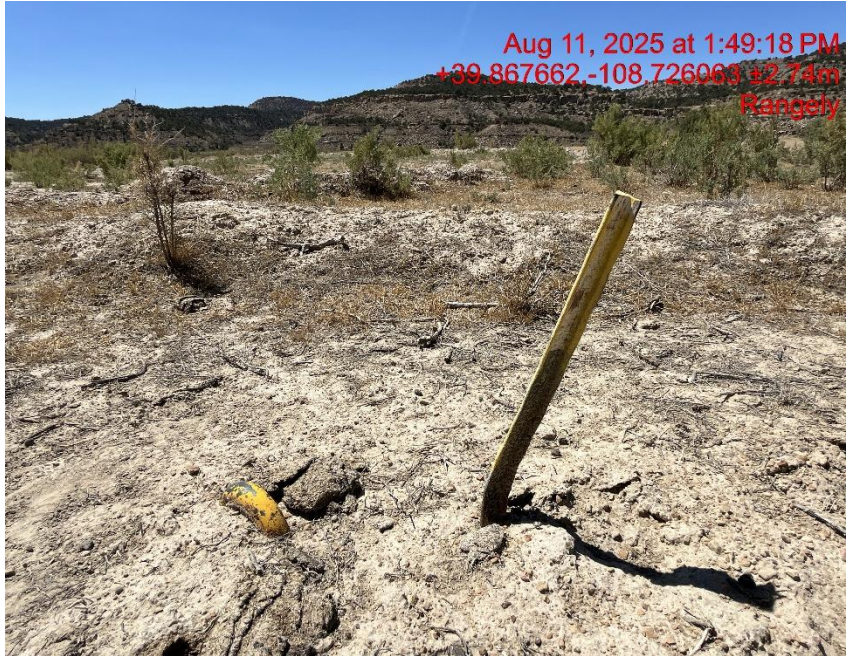
Photo # 1722 Improperly marked deadman
