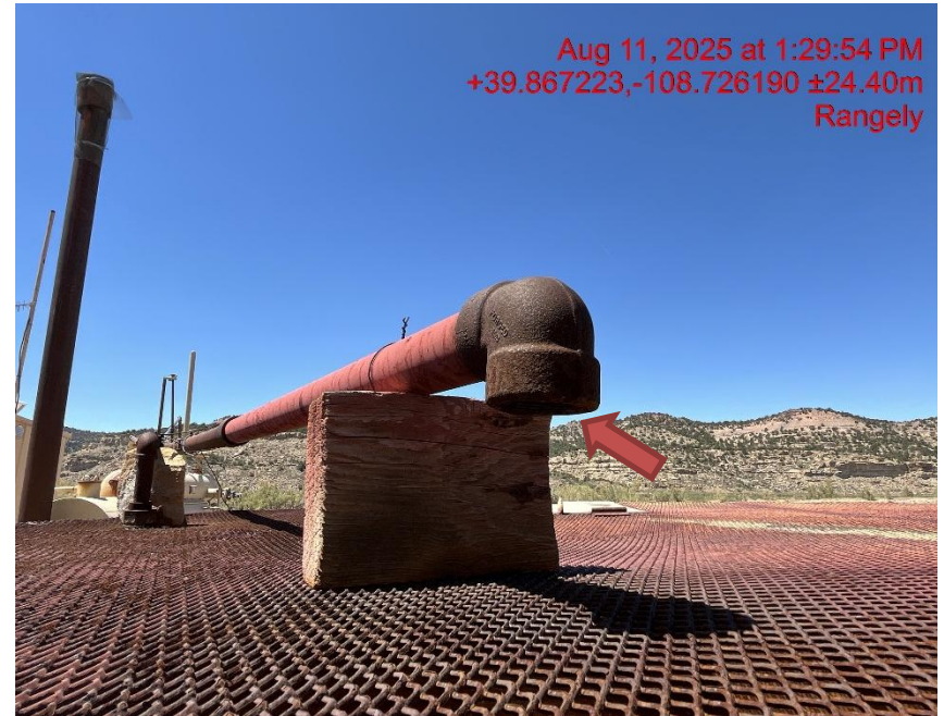
Photo # 1710 Open ended piping/wildlife hazard/available for entry by wildlife
