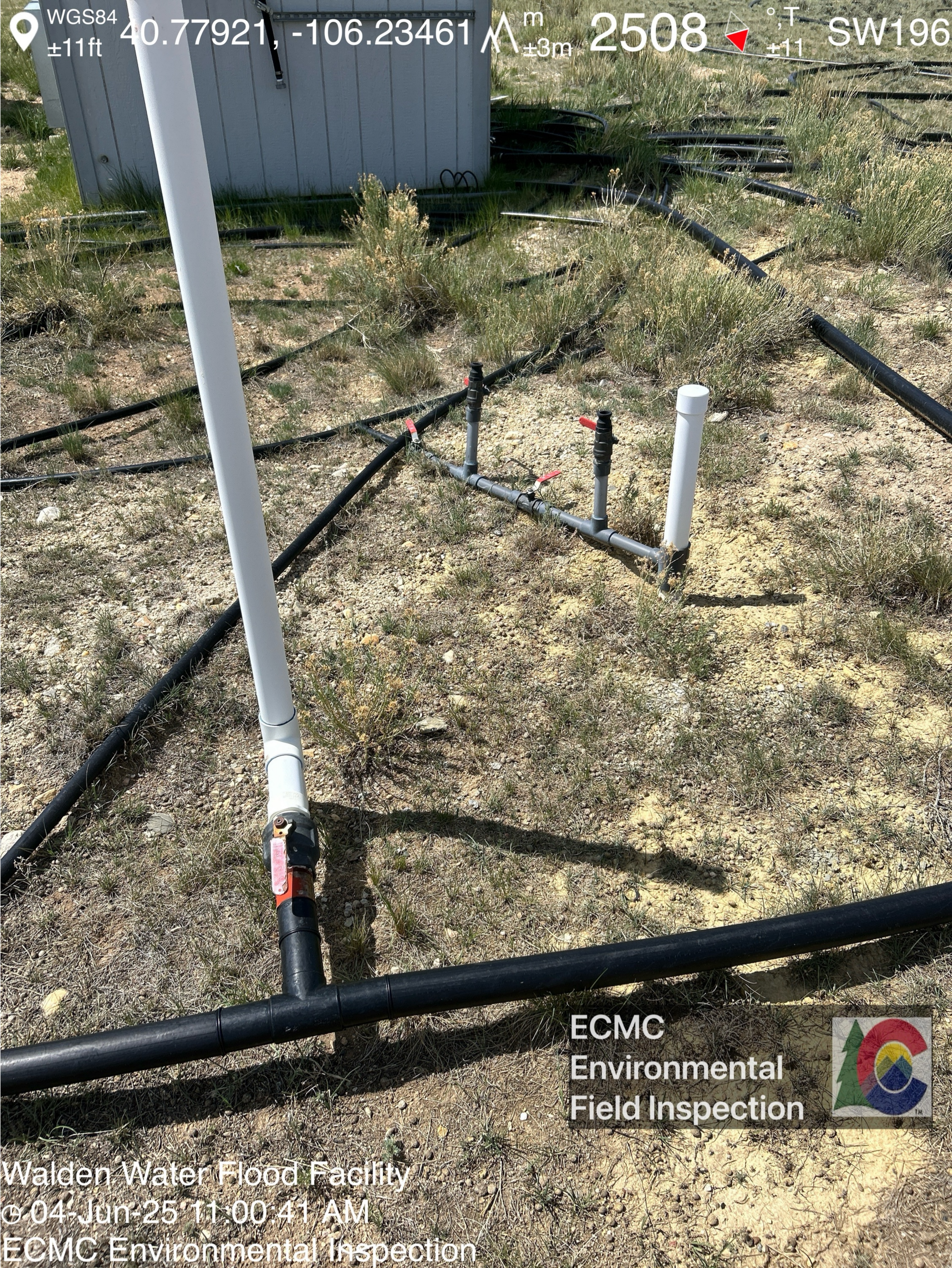
Looking at above-ground conveyance line manifolds.
