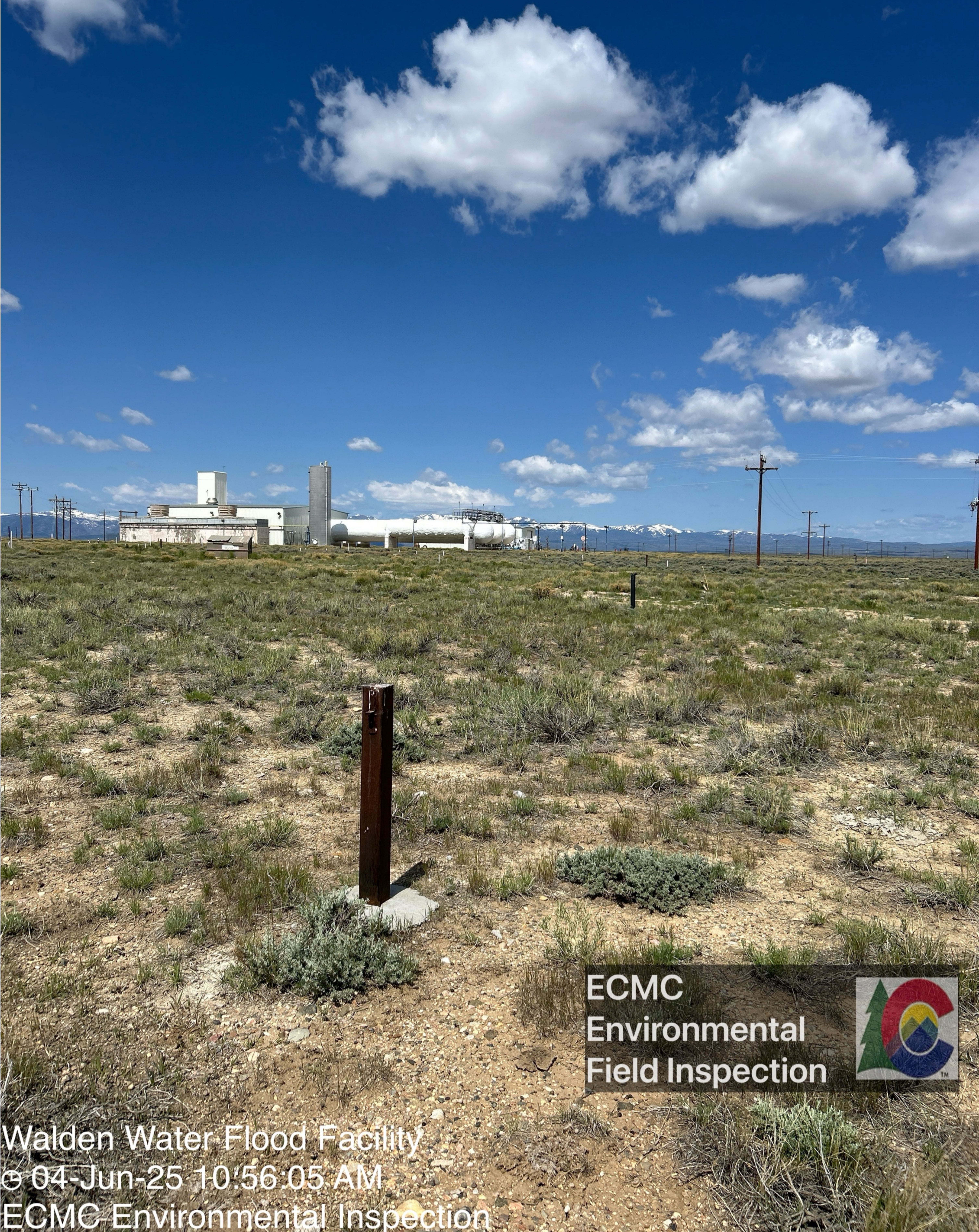
Looking west at the network of monitoring wells and air sparge/soil vapor extraction system wells. Metal monitoring well monuments are visible.
