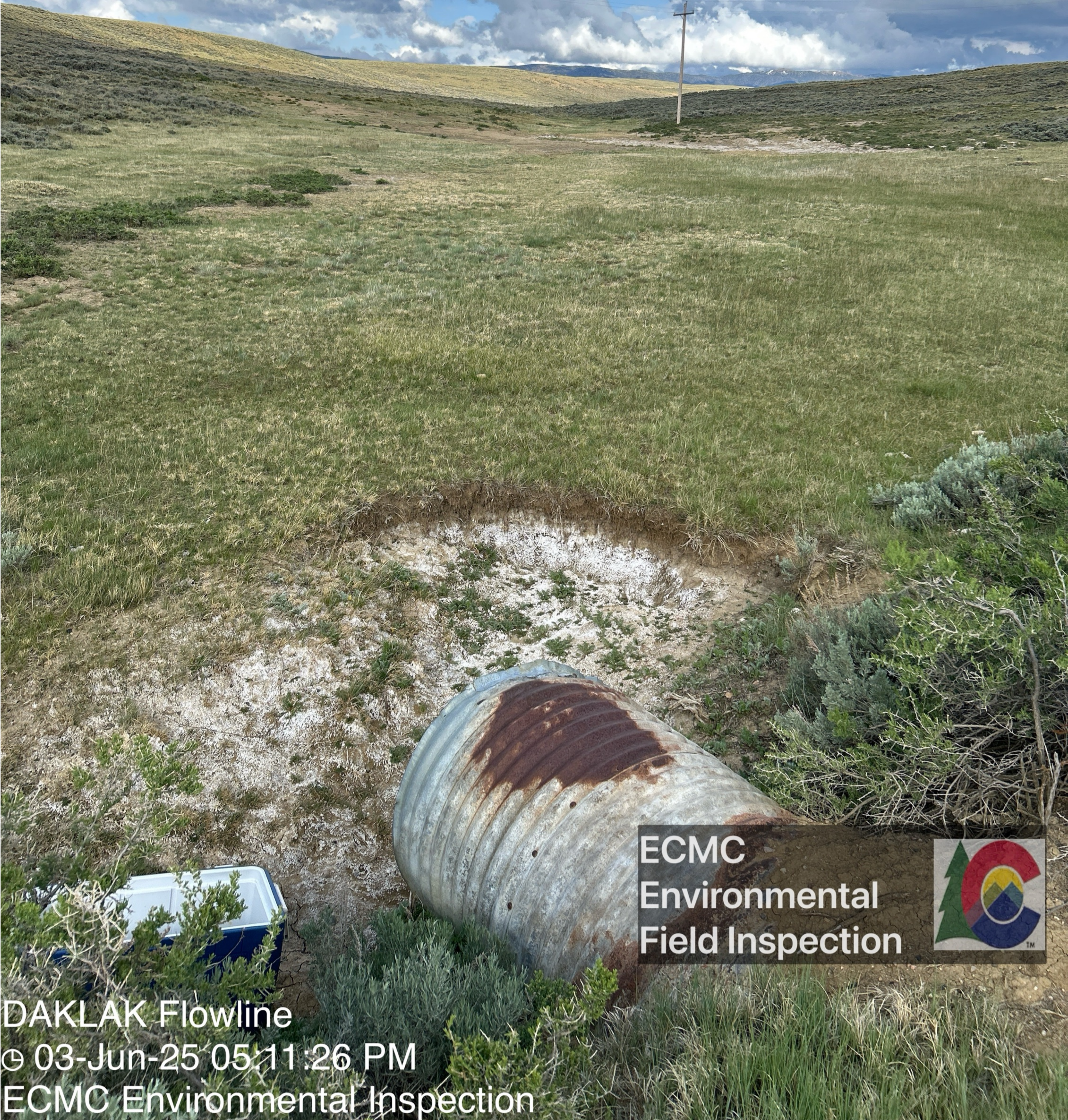
Looking at drainage towards spill location. Trash (a cooler) and salt crusting are visible adjacent to a culvert running under the access road.
