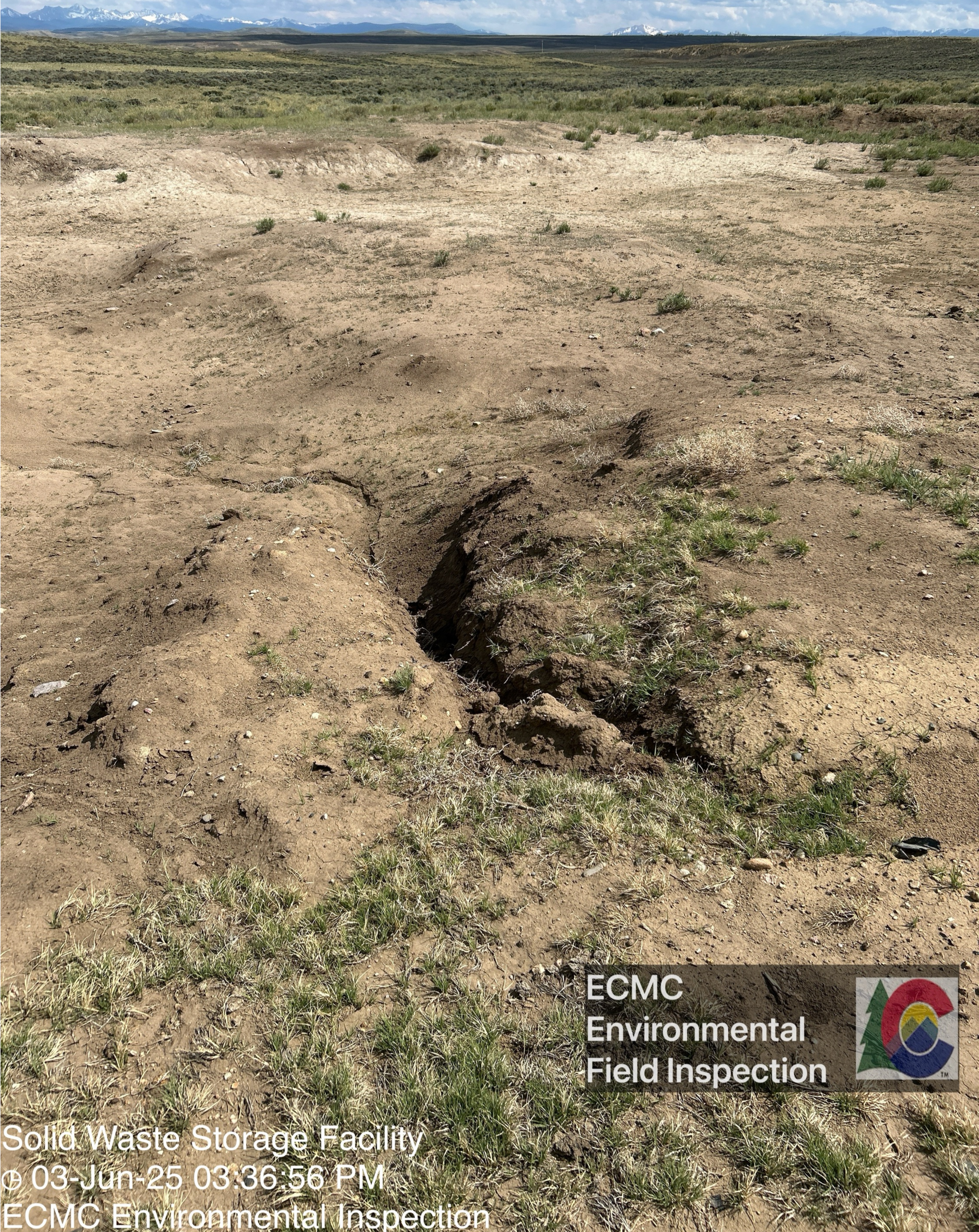
Rill erosion is visible along portions of the sidewalls of the excavation.
