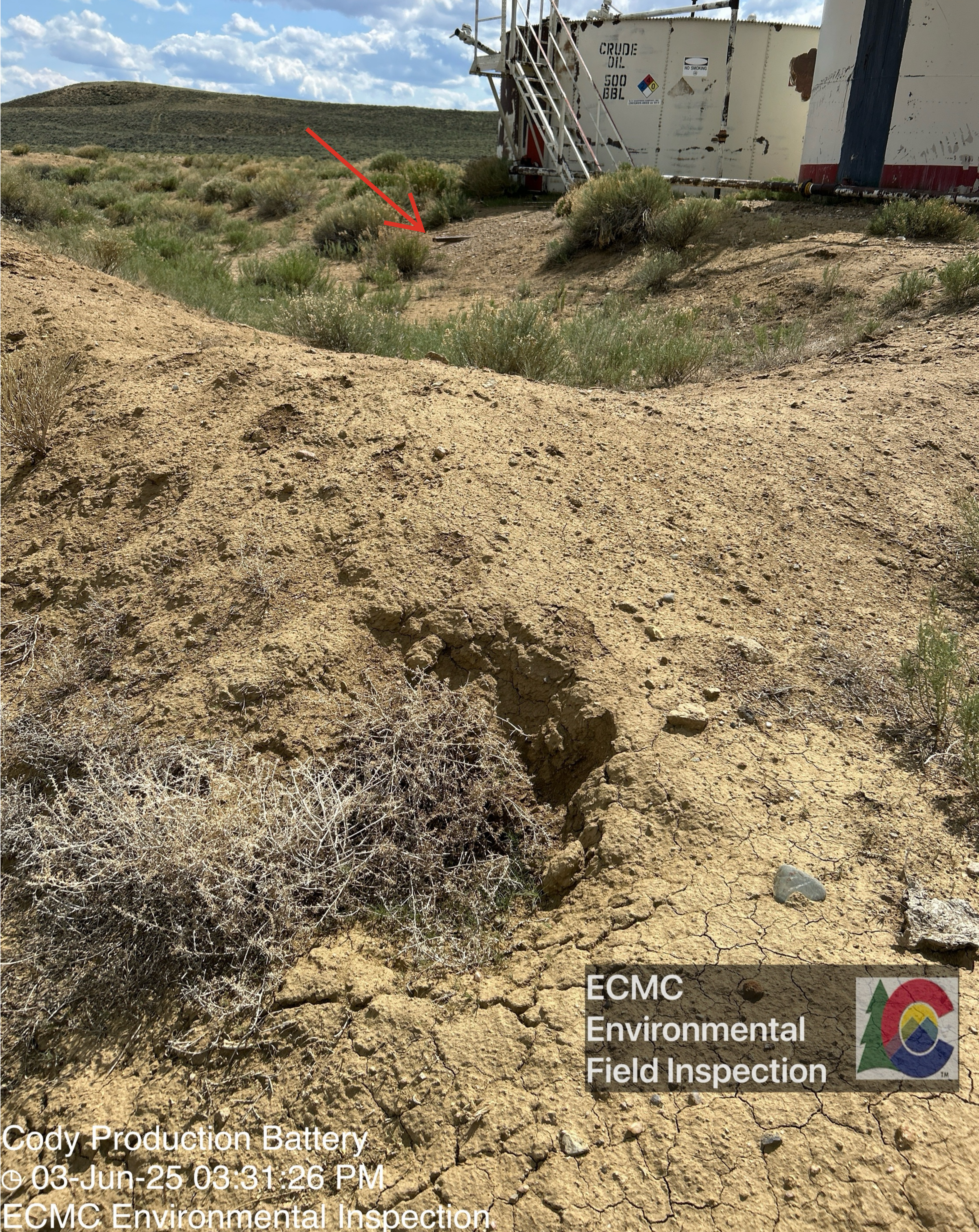
A metal pipe is visible protruding from the berm adjacent to the production tanks. Holes, debris, and weeds are visible on the berms.
