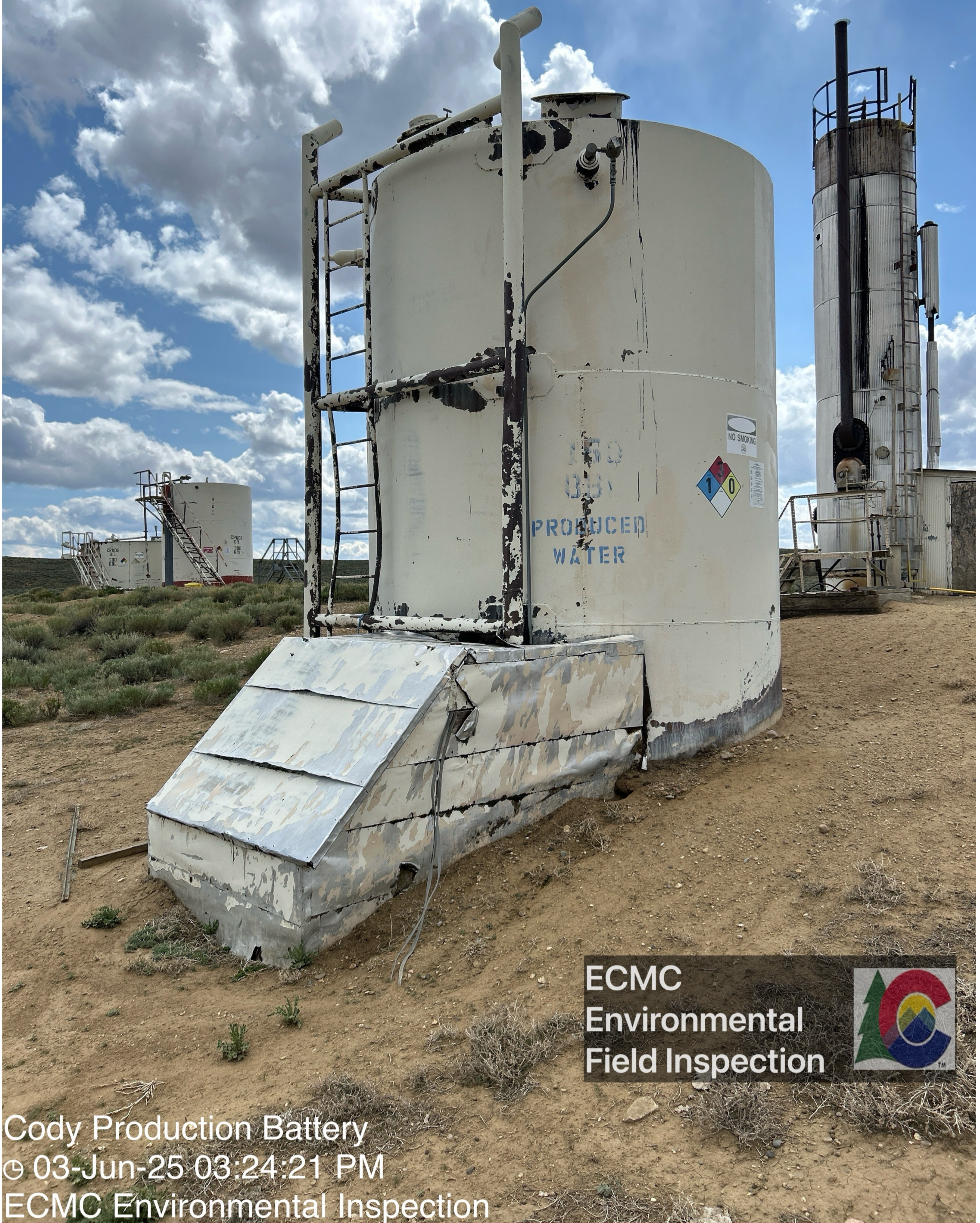
Labels/placards on a produced water tank are becoming illegible.
