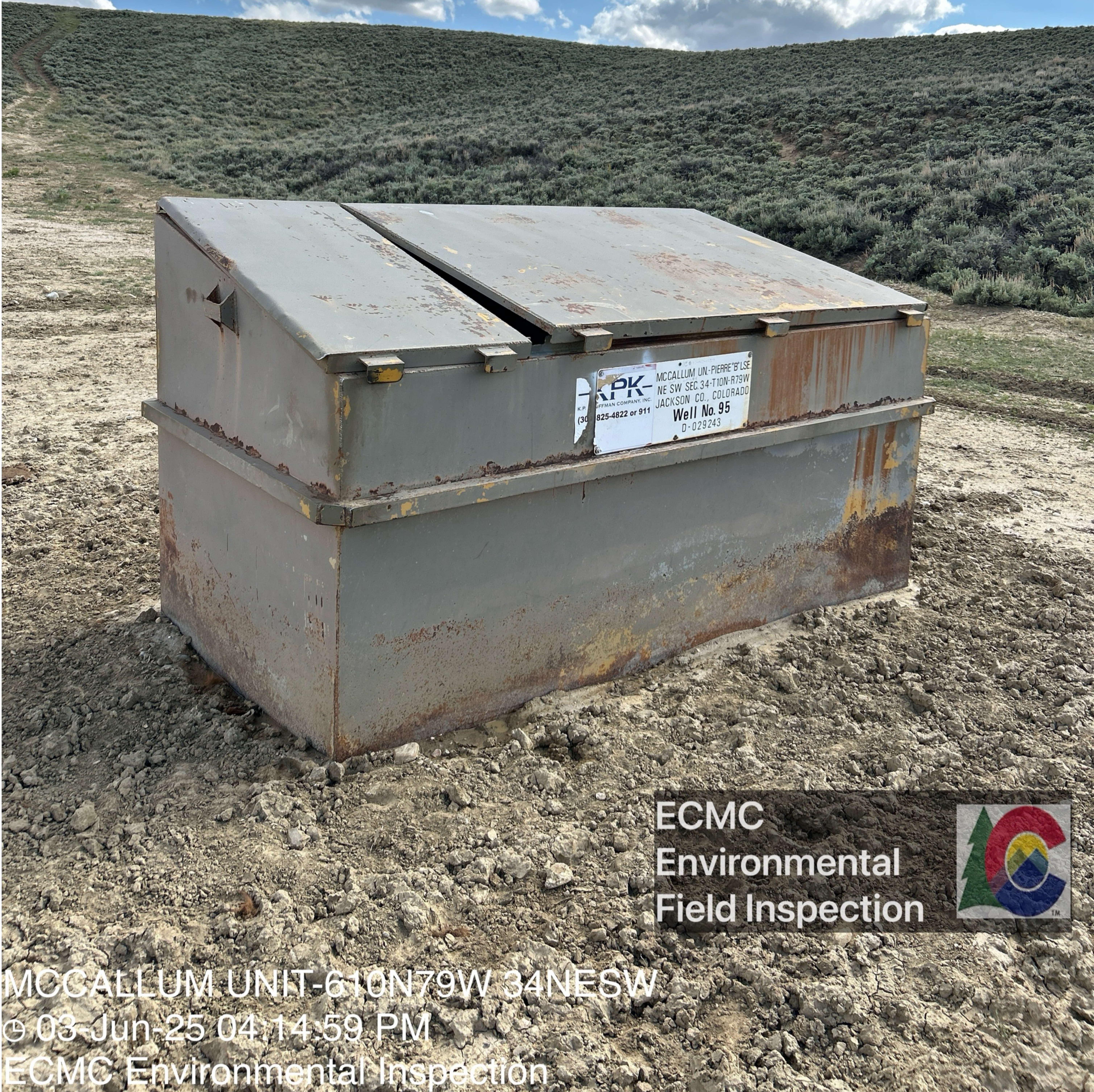
Signage with emergency contact number is peeling and becoming illegible at the MCCALLUM UNIT-610N79W 34NESW well.
