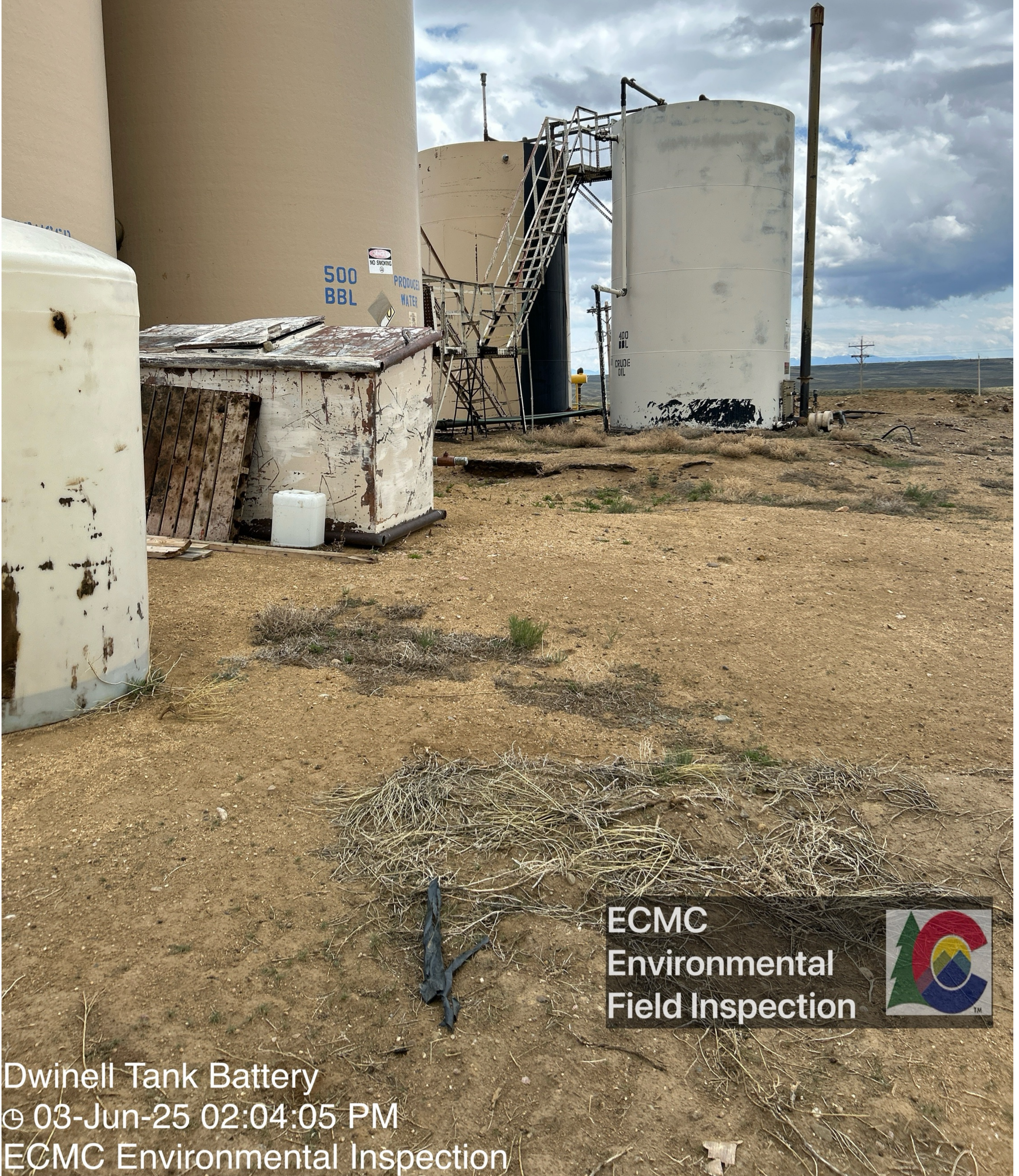
The placard on a produced water tank has peeled and is illegible. Weeds and trash are visible on location.
