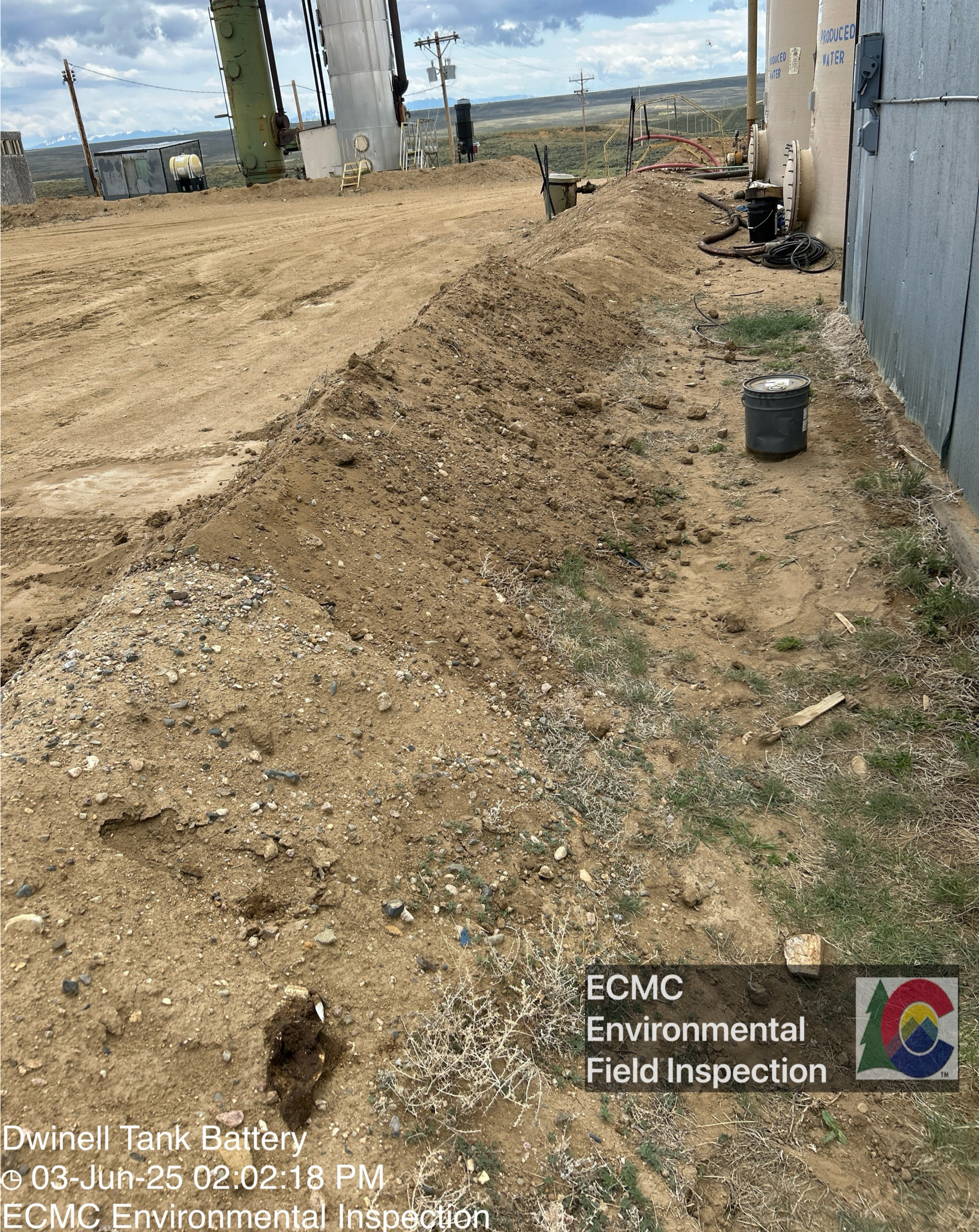
A portion of the berm appears to have been recently repaired; however, the berm does not appear to have been consolidated.
