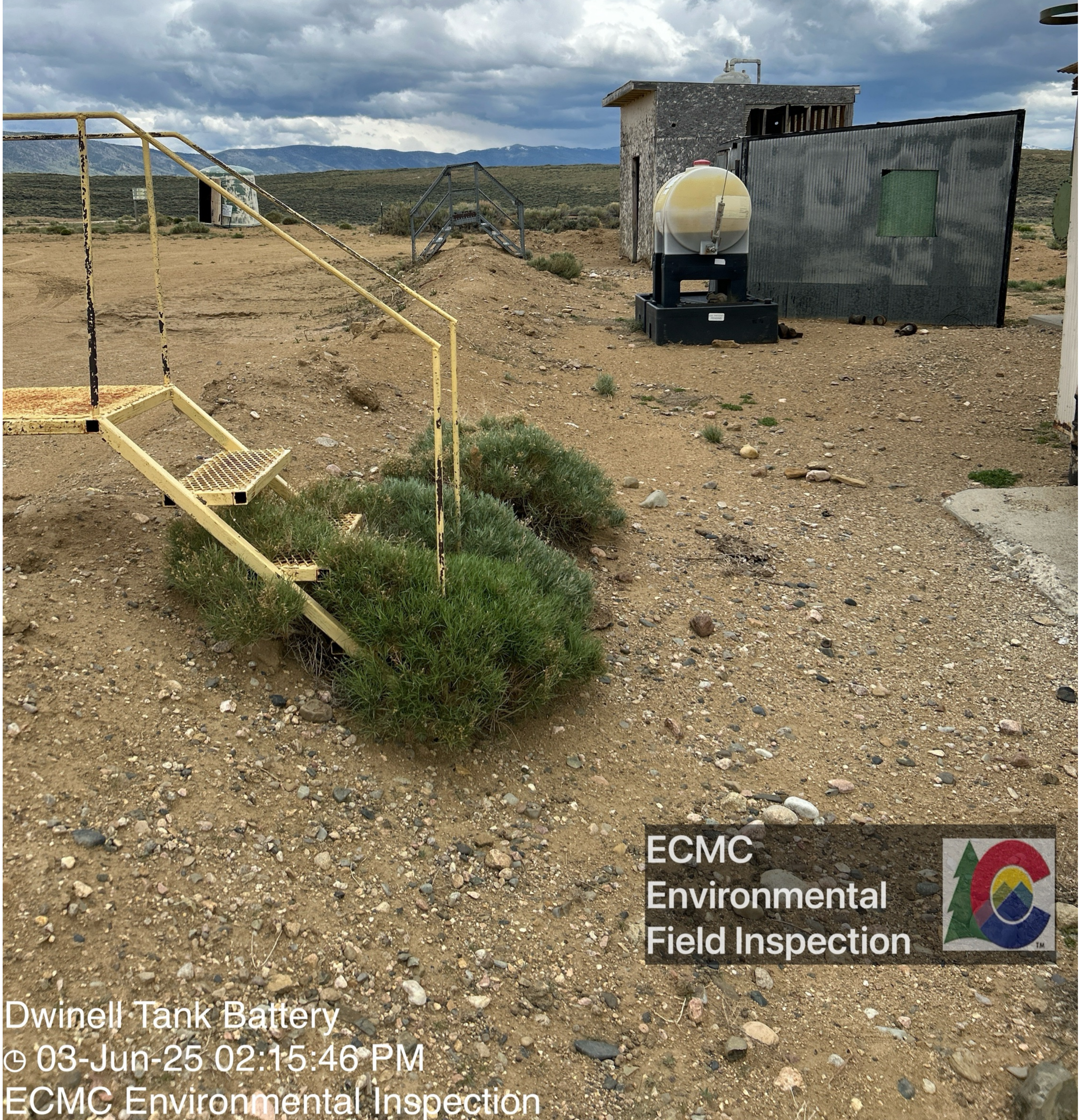
Looking at the separator equipment containment berm. Portions of the berm appear to have been eroded.
