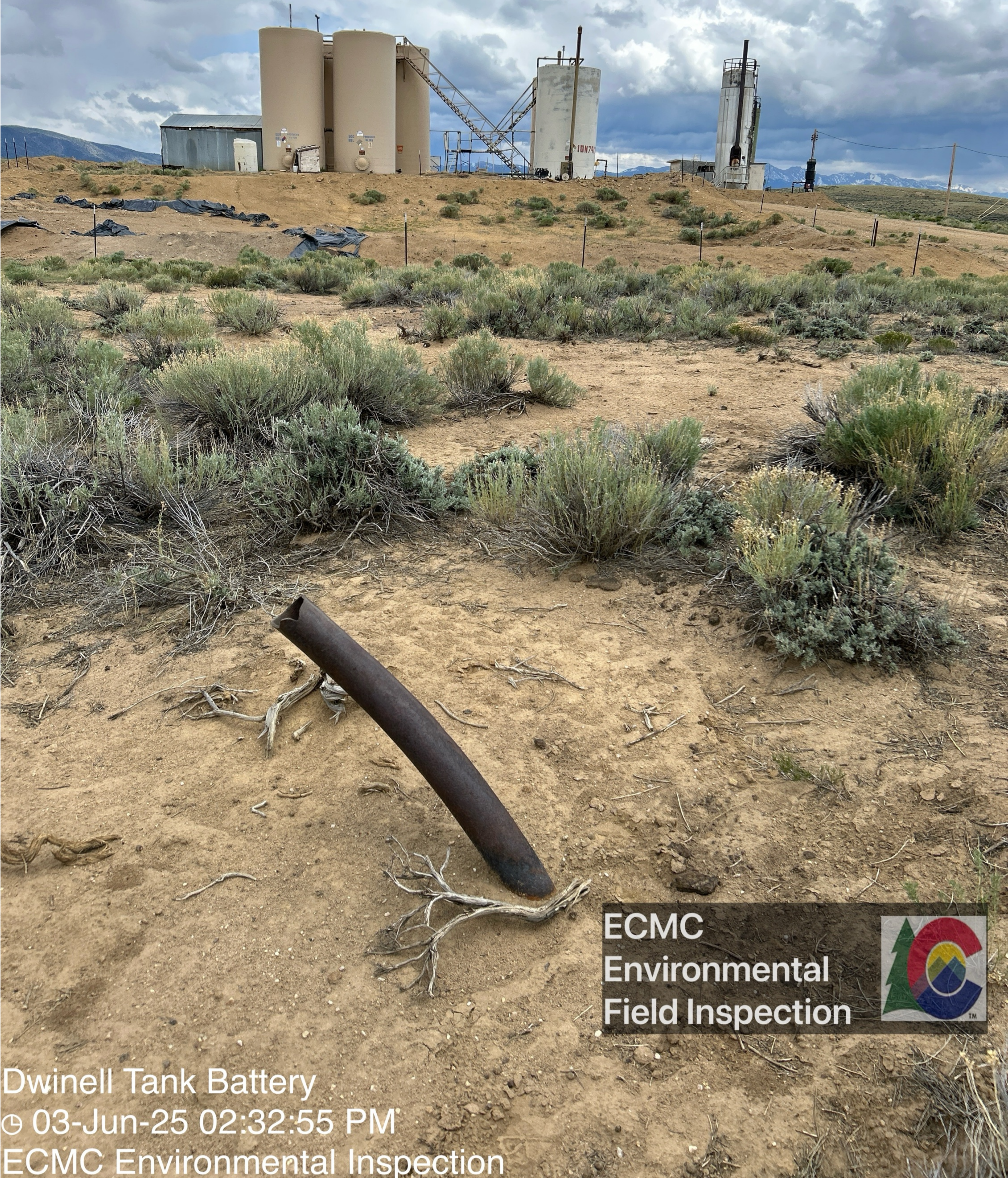
A metal line/riser is visible protruding from the ground surface west of the location.
