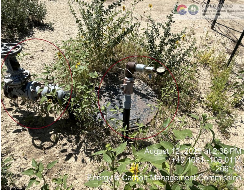
Unmarked Risers/ Overgrown vegetation
