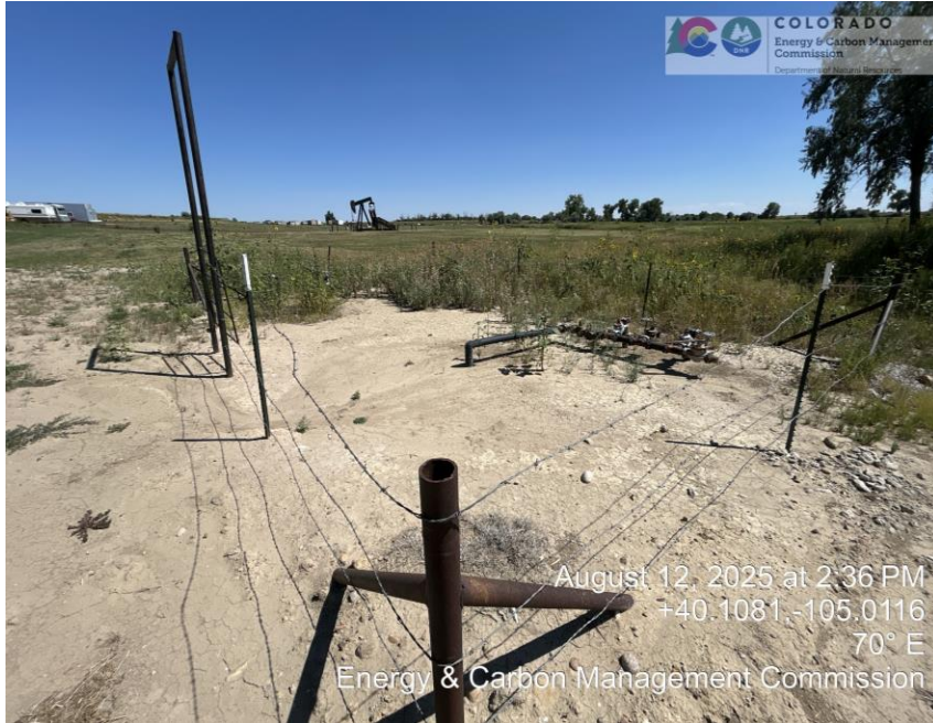
Header Location/ overgrown vegetation
