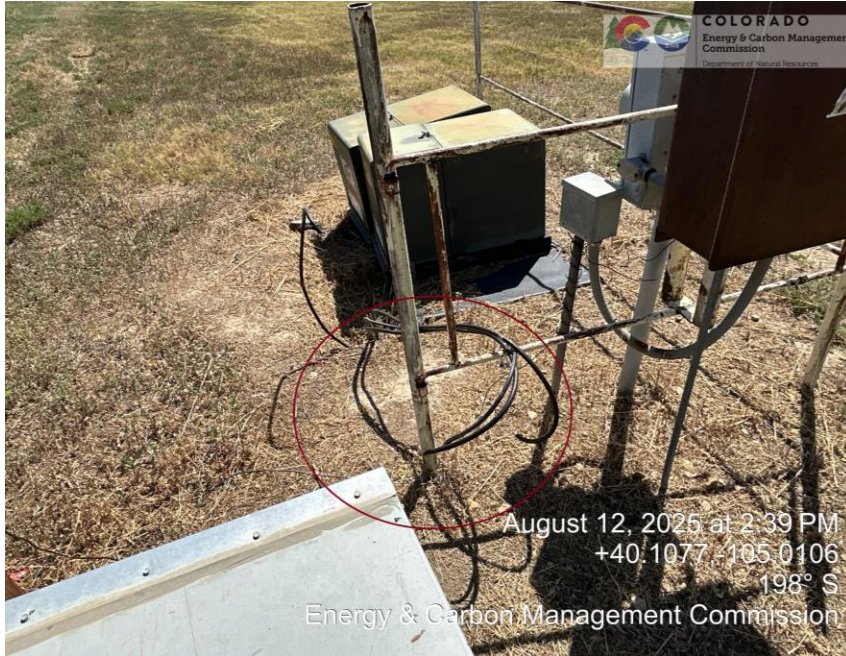
Exposed wires for pumping unit electrical box/ transformers appears to be a safety hazard.
