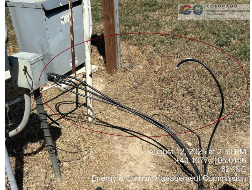
Exposed wires for pumping unit electrical box/ transformers appears to be a safety hazard.
