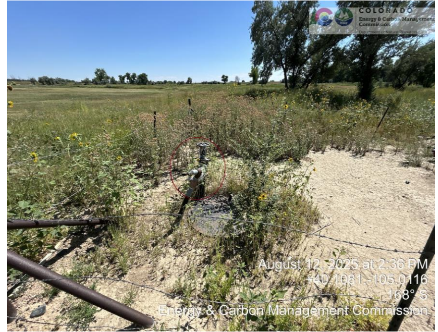
Unmarked Risers/ Overgrown vegetation
