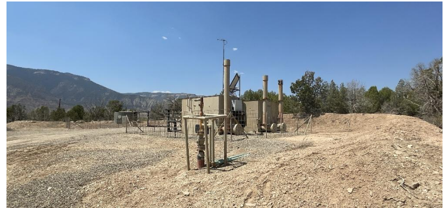
South East corner of location.
