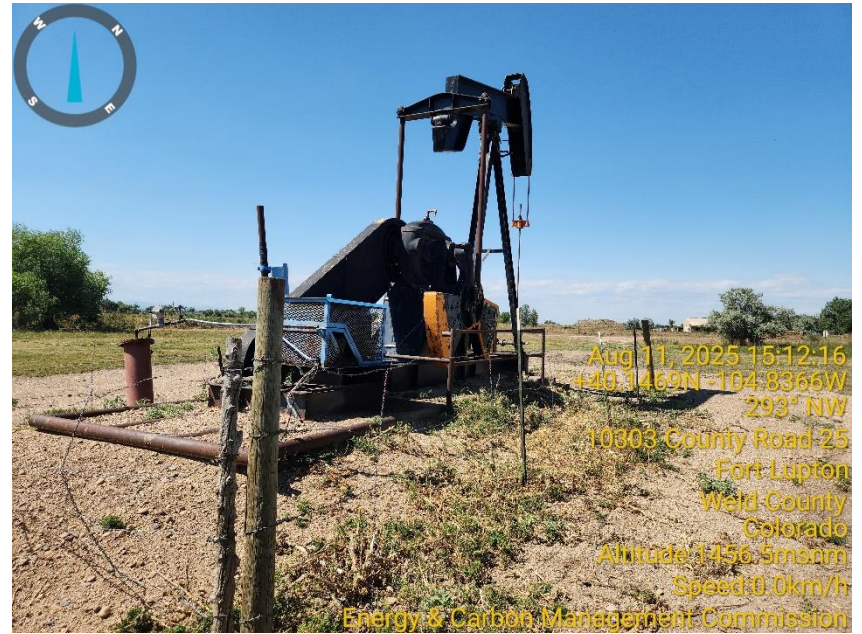
Photo 4 Gas engine/Pump jack.
