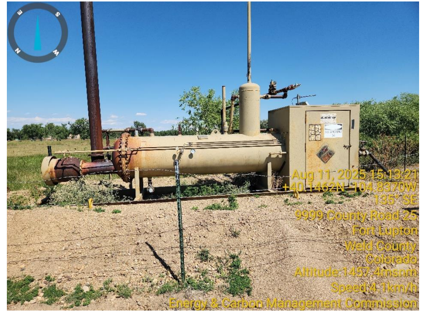
Photo 8 Horizontal Heated Separator.
