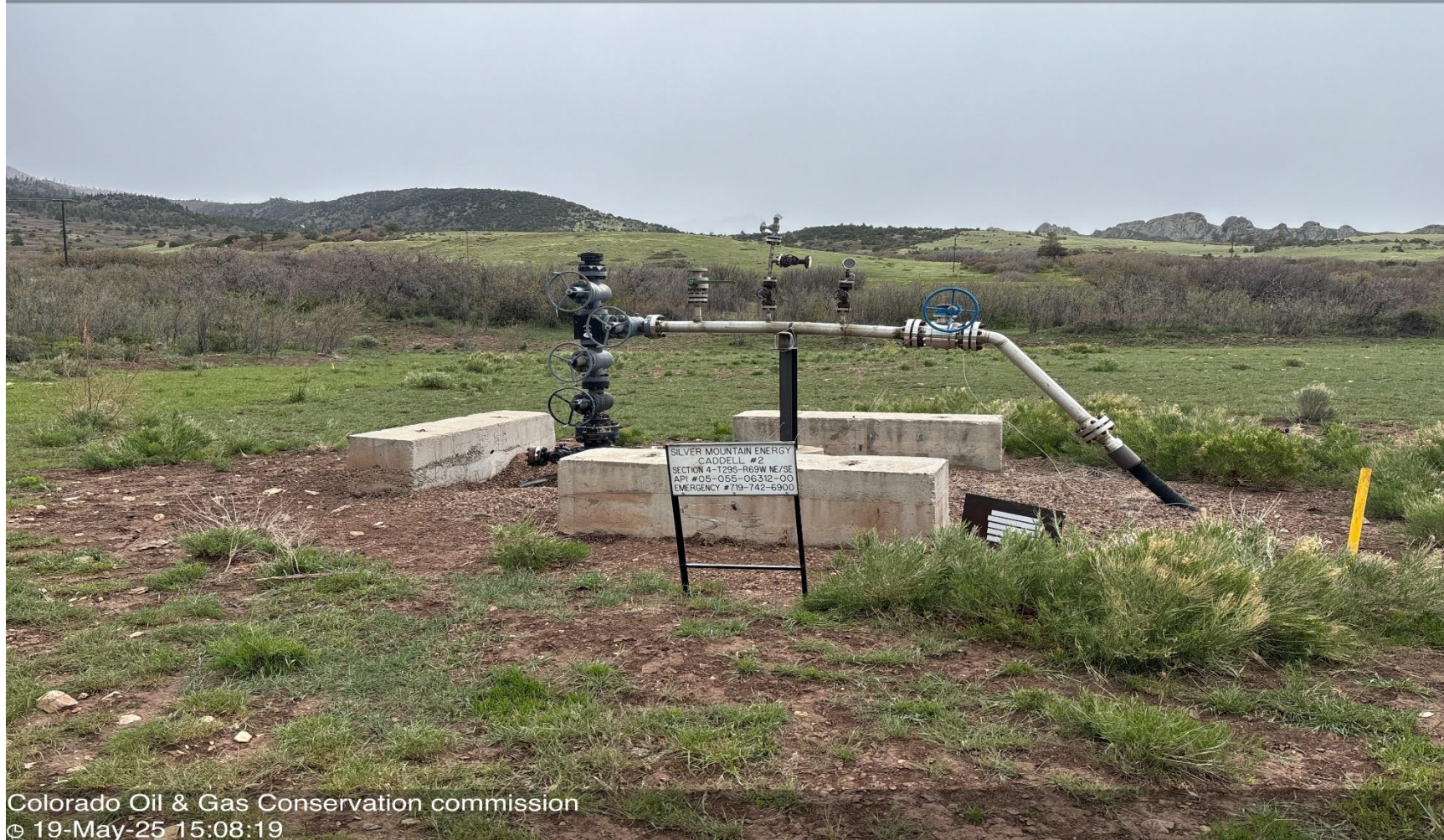
PHOTO 6: WELLHEAD AND EQUIPMENT.
