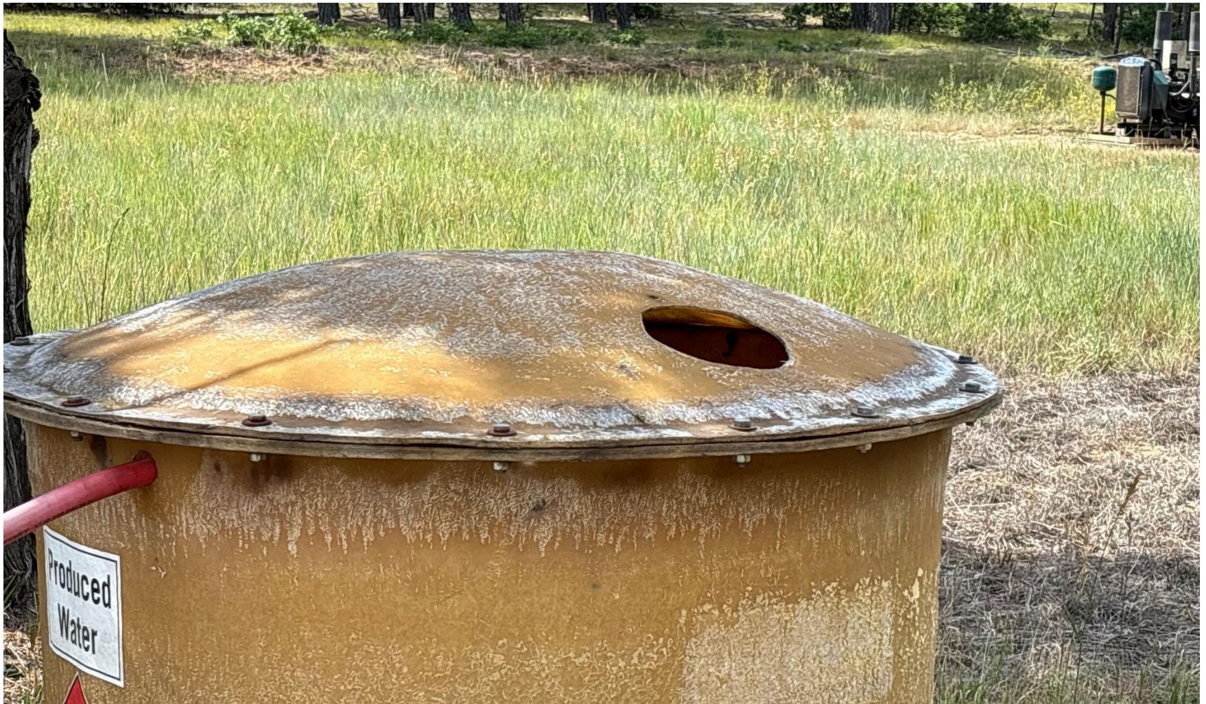
PHOTO 4: PRODUCED WATER TANK AT THE ENTRANCE OF LOCATION HAS A HOLE IN THE TOP THAT IS NOT COVERED. Install or repair wildlife protection equipment. CA DATE 8-22-2025.
