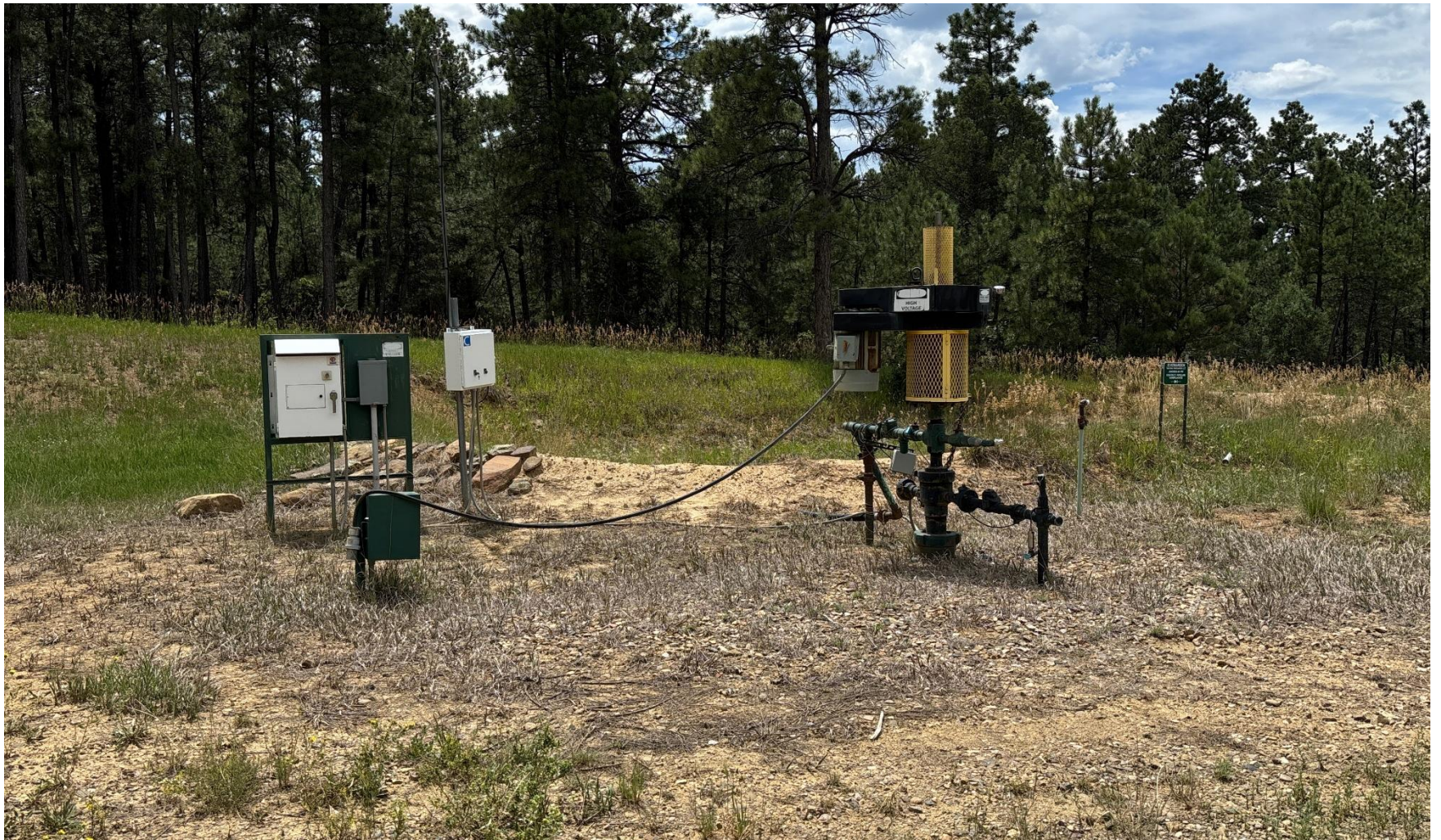
PHOTO 3: WELLHEAD AND EQUIPMENT.
