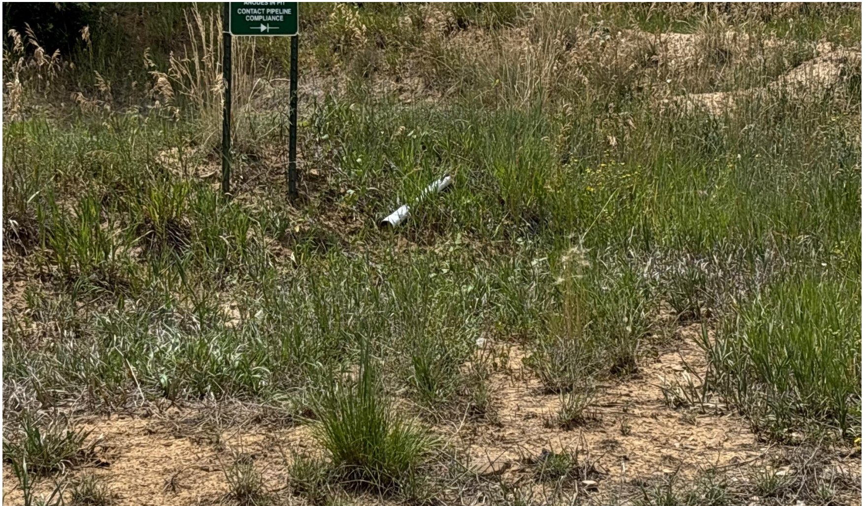
PHOTO 7: WEEDS ARE STARTING TO ENCROACH NEAR WELLHEAD. MAINTAIN WEEDS PER RULE 606. CA DATE 8-22-2025.
