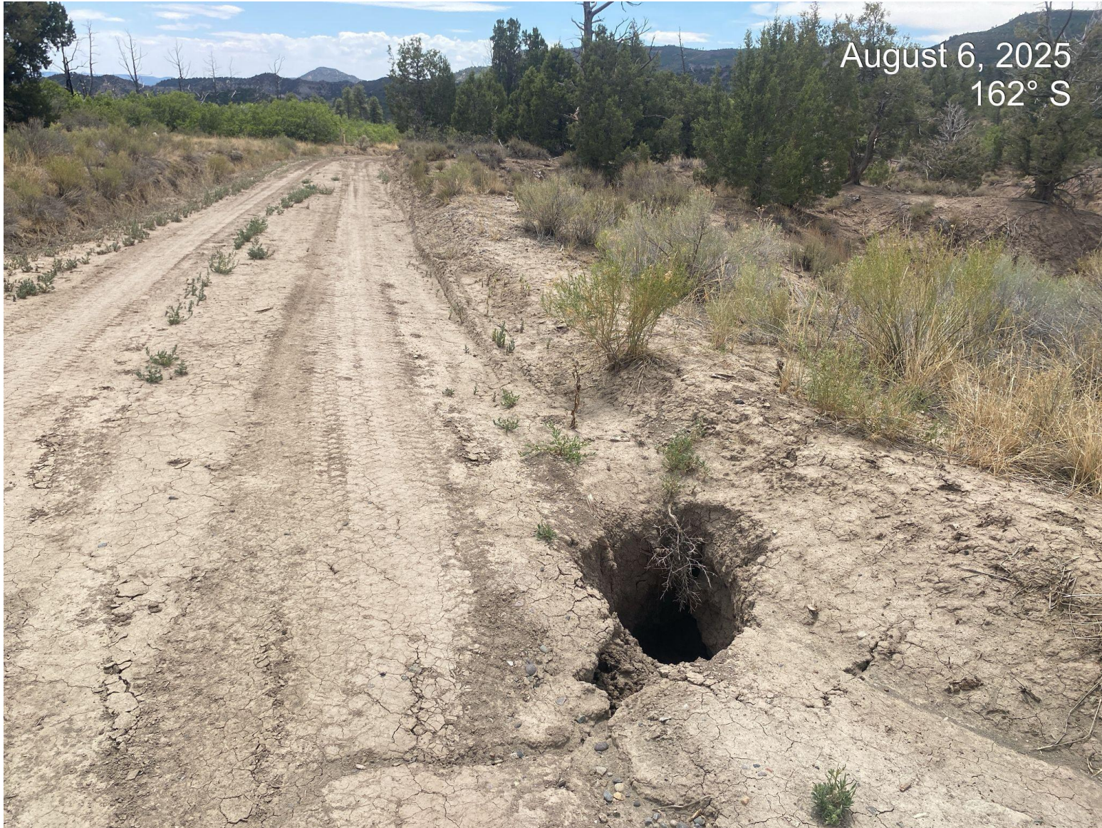
Photo 3. Erosion/tunnelling occurring at location access point.
