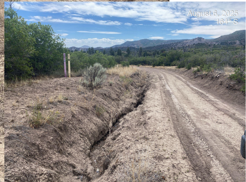
Photo 5. View of drainage adjacent to access road that has not been installed per good engineering practices, BMPs are missing and runoff along the access road drainage is resulting in degradation and incising.
