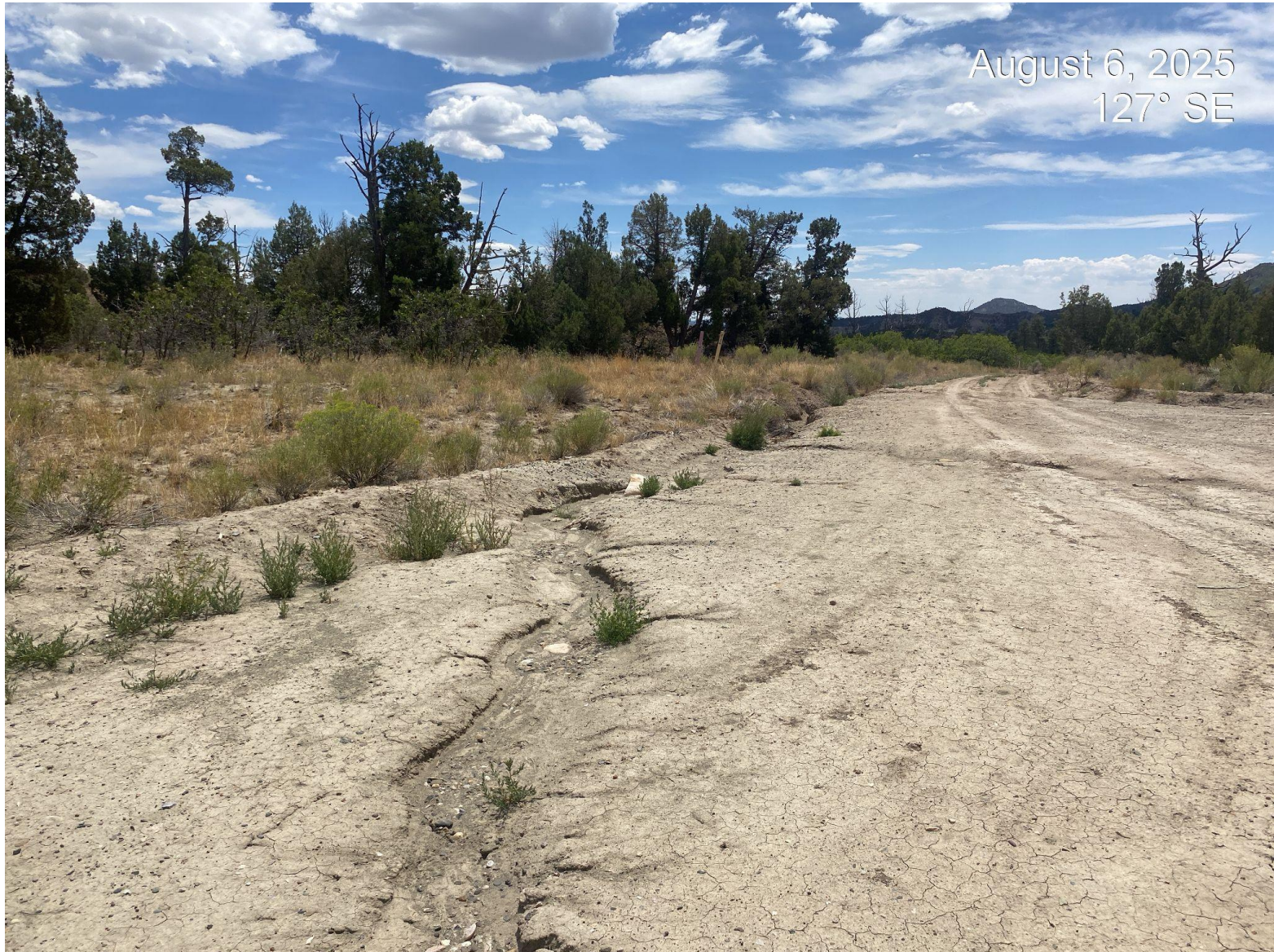
Photo 2. Erosion occurring at location access point.
