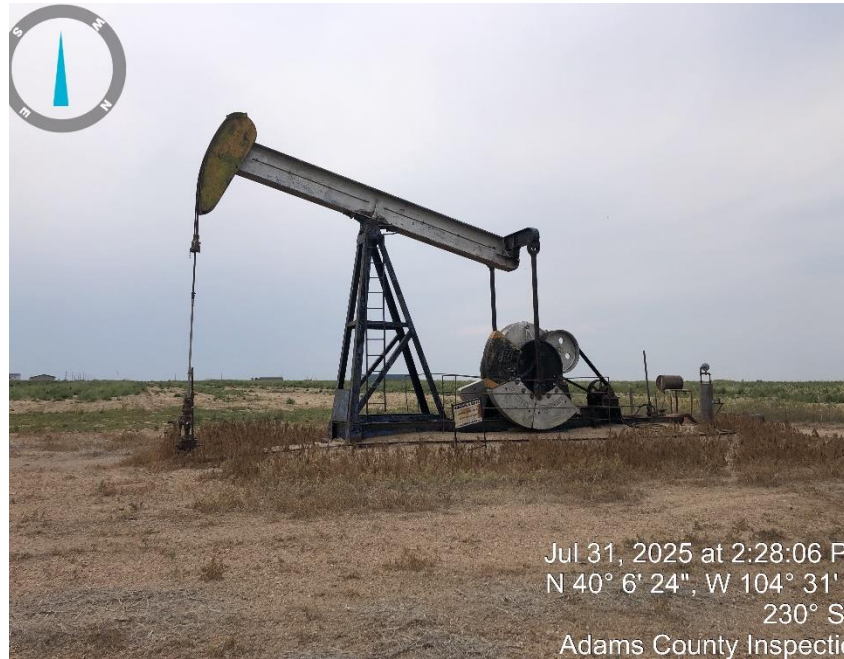
Photo #1 Pump jack.
