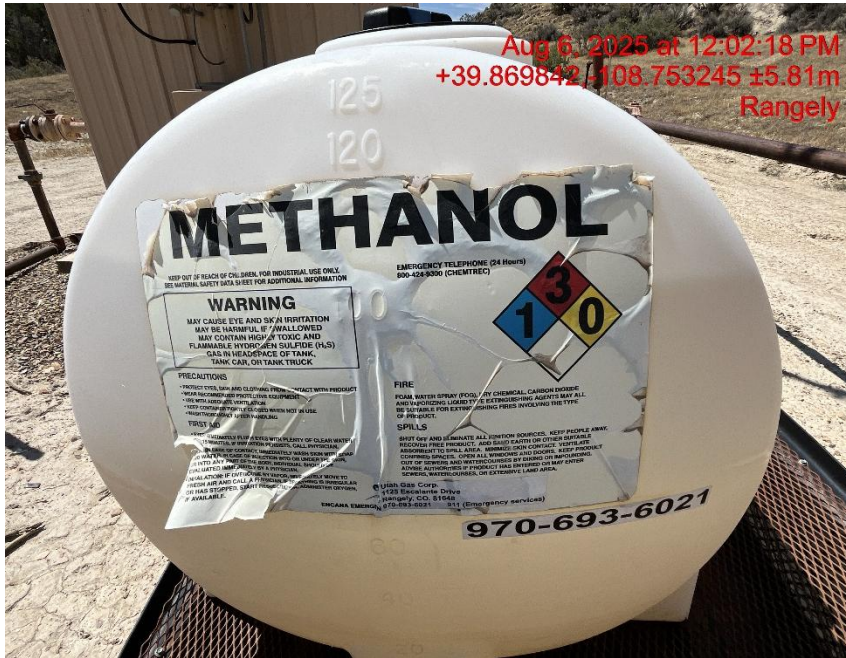
Photo # 1409 Chemical tank label is weathered and peeling
