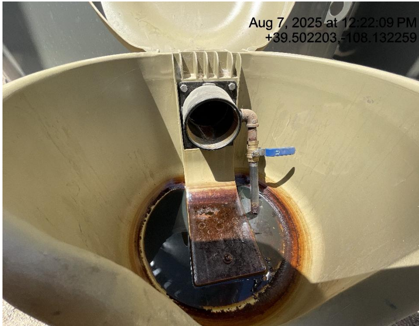
Photo # 9195 Open ended load line
