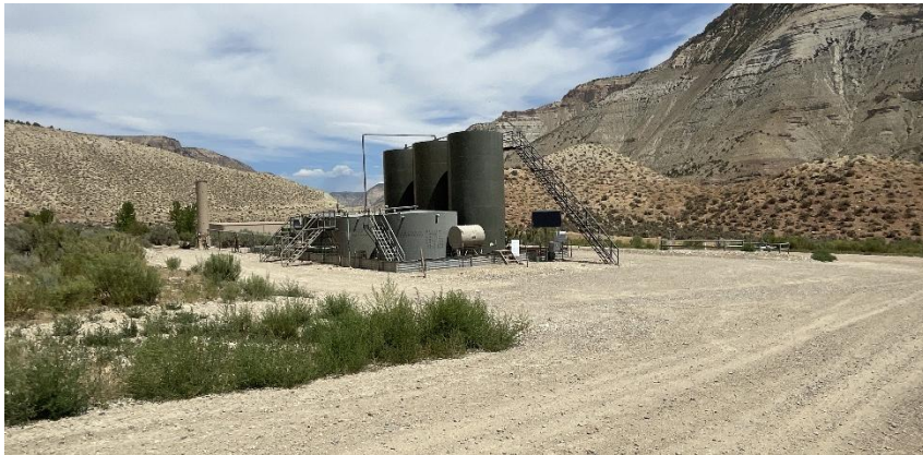
South West corner of location.
