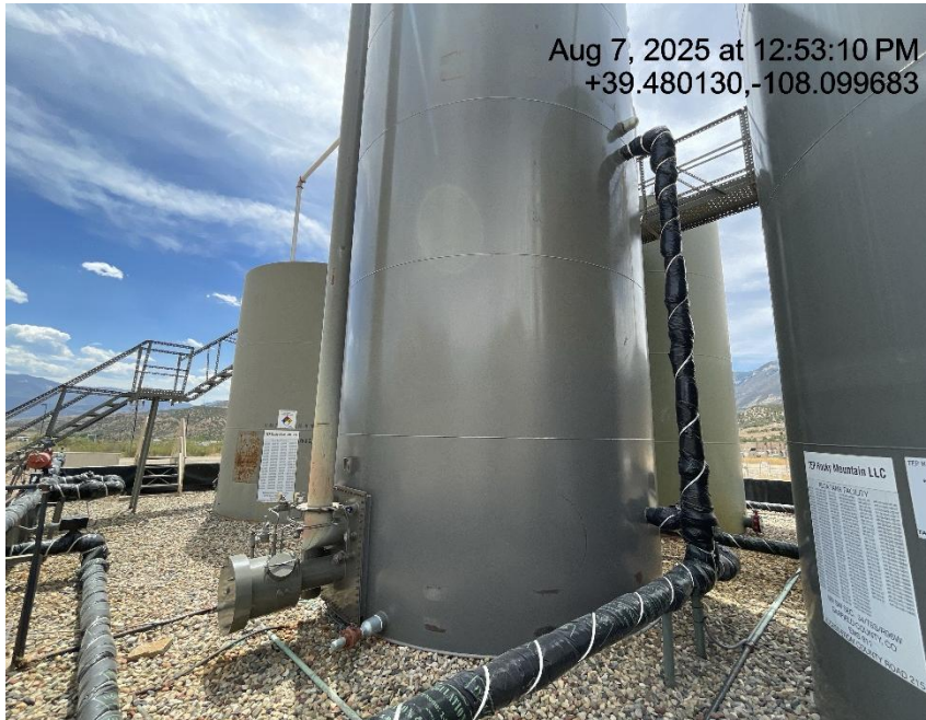
Photo # 9301 Tank lacks required labeling
