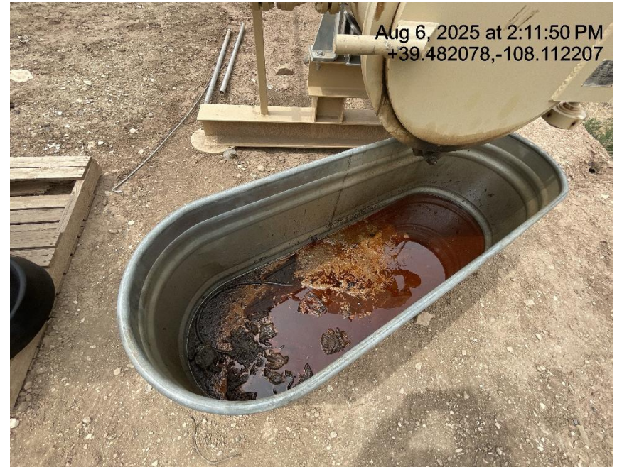
Photo # 8562 Containment near pig station contains unknown fluid & is available for entry by wildlife/wildlife hazard
